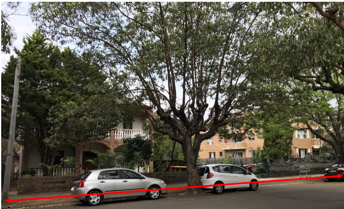
Picture 2: Subject site viewed from Tintern Road.
