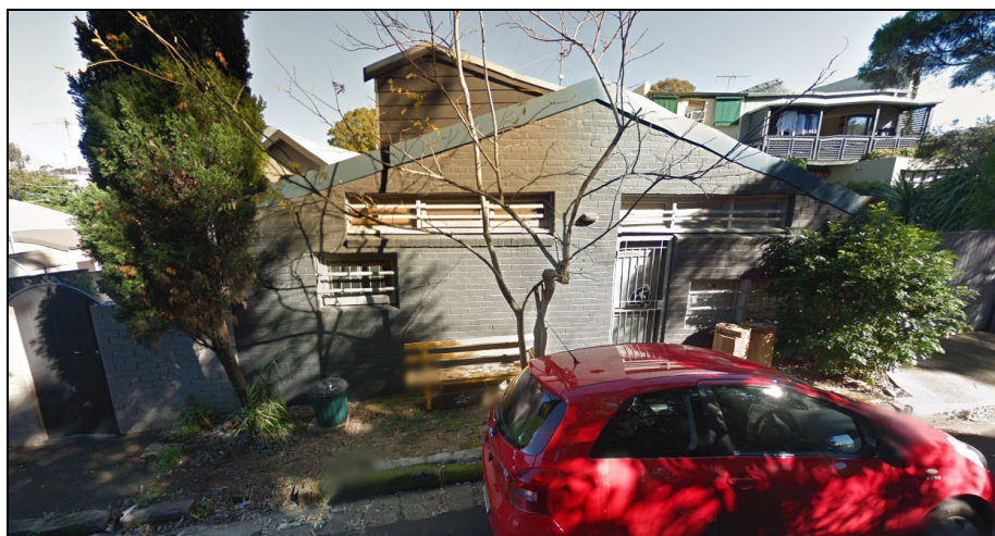
Figure 1: Front elevation of dwelling from Emily Street. Source: Google streetview.
