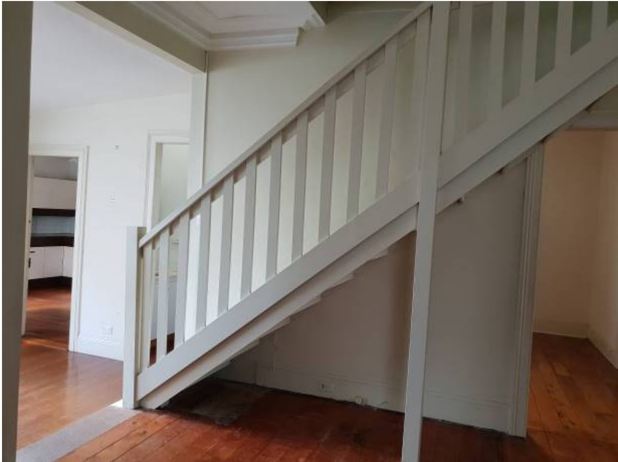
Figure 5: Photograph taken during site inspection (4 September 2018). Note the new internal staircase and new wall opening.
