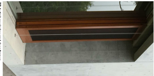
TB-1: timber window and door frames, ground floor addition
