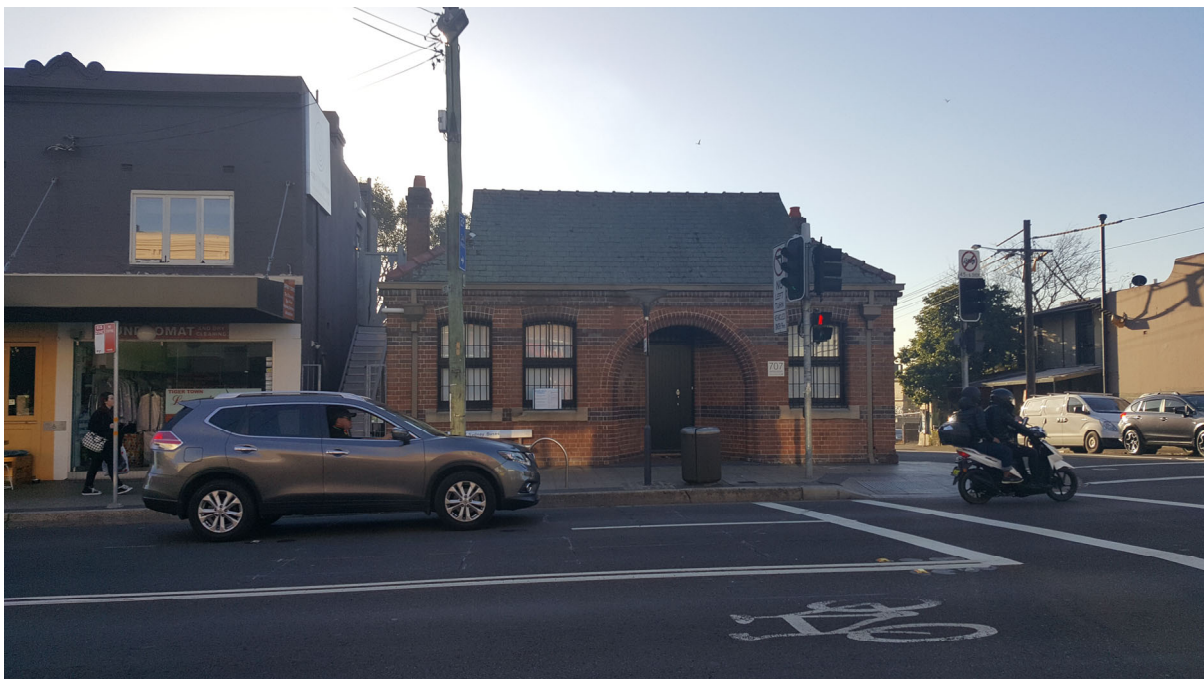
Figure 2 – View of the subject site from Darling Street
