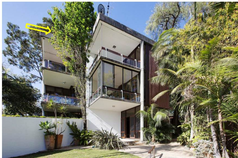
Figure 4: Quercus robur (English Oak), showing limited canopy spread due to proximity to the building. Source: Brian McDonald
