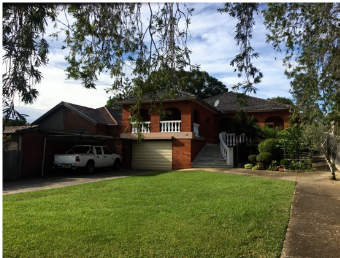
Figure 1 47 Wolseley Street Haberfield – View from front boundary
