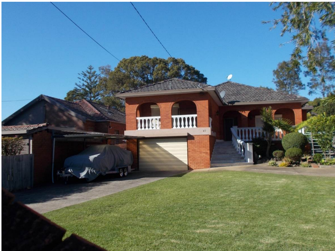
Picture 2 Site Photo – Wolsley Street frontage
