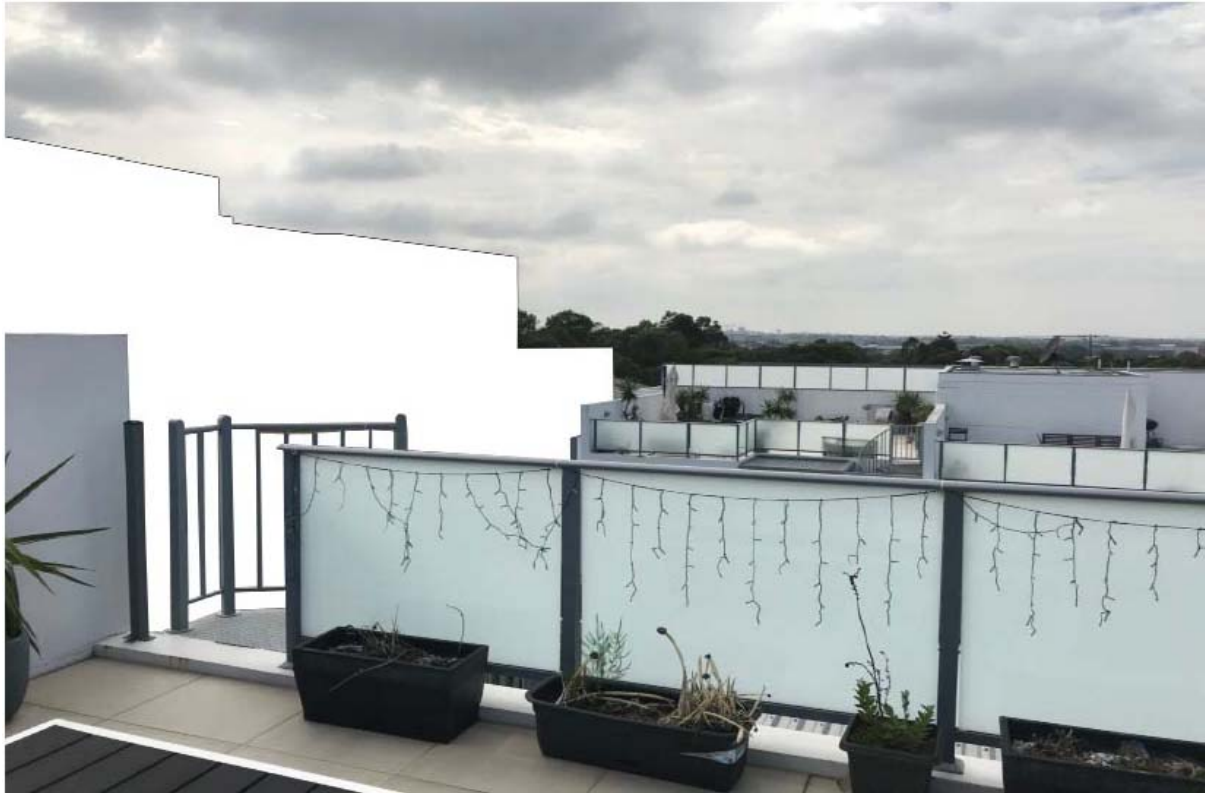
Picture 10 – View north east from the roof terrace at unit 28 – showing the building envelope conditioned by the Inner West Local Planning Panel.
