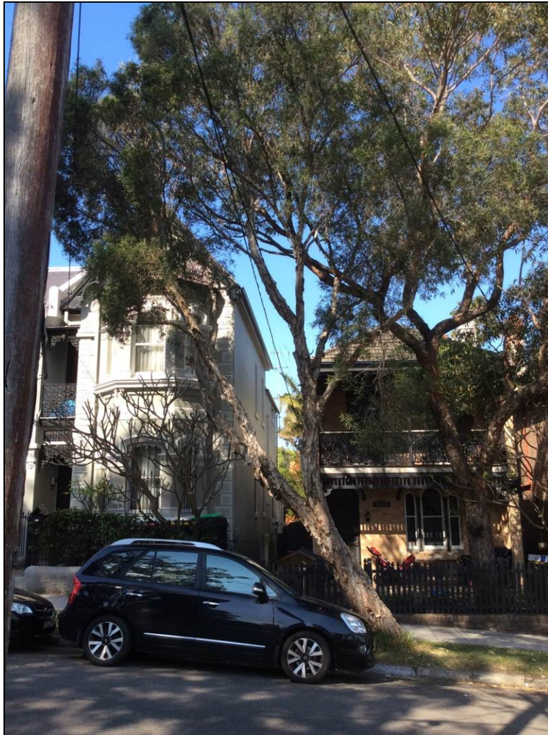
Image 2: Southern side of dwelling and area of addition as viewed from the street
