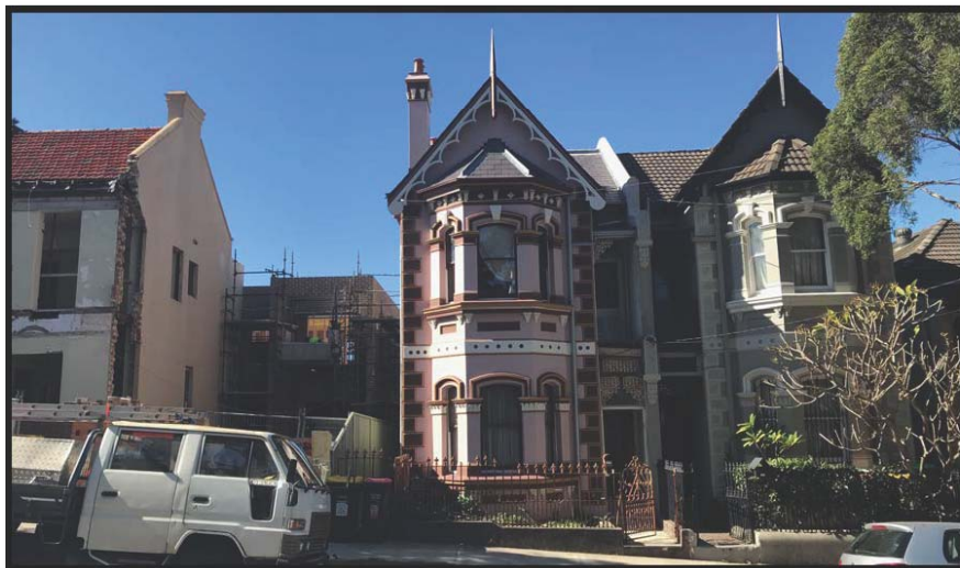
Photograph 2 – View of site (right) from John Street
