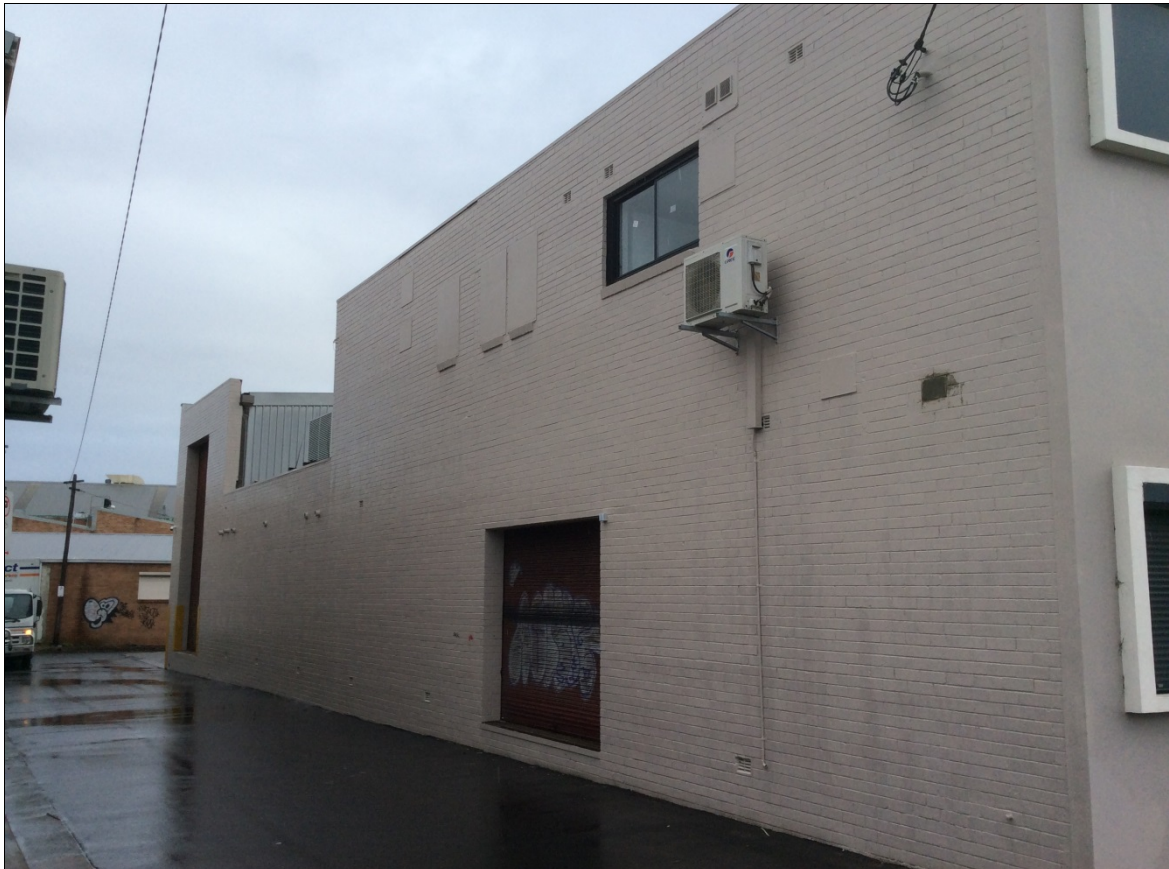
Image 2: View of the eastern elevation at Buckley Lane
