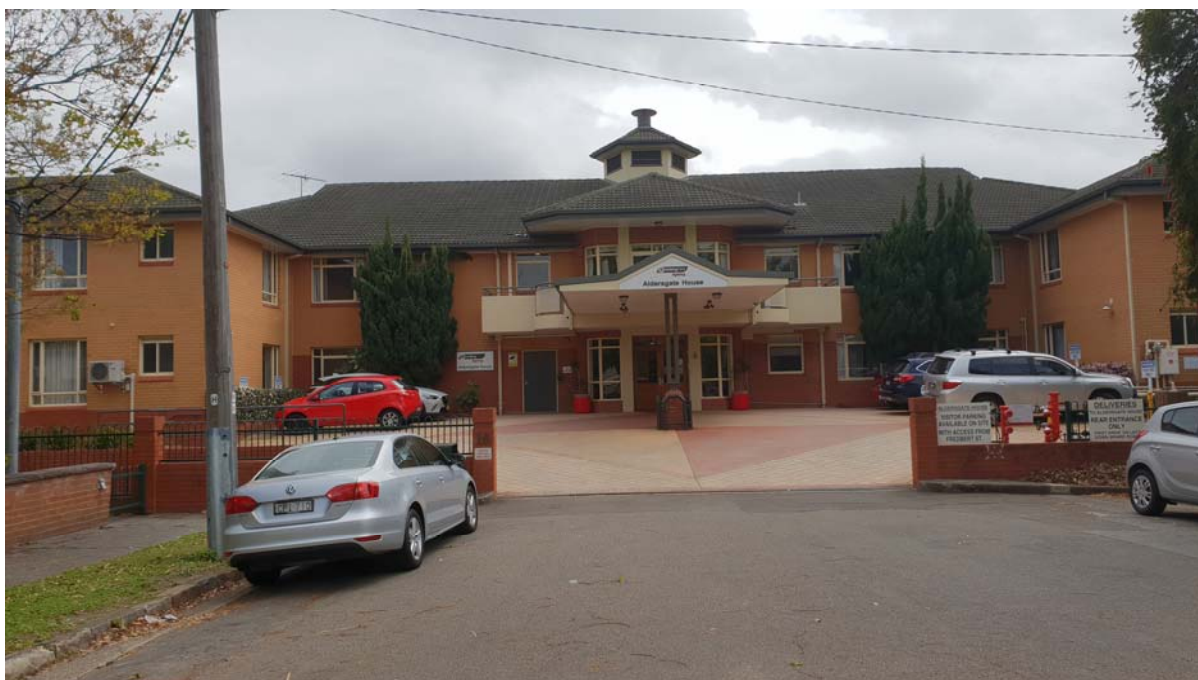
Figure 2: Fredbert Street frontage
