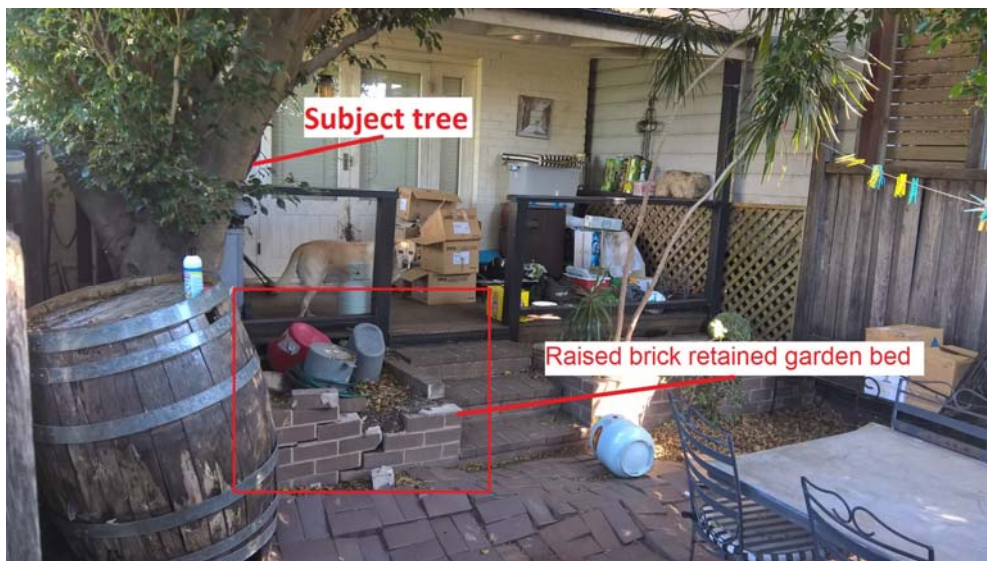
Figure 4: Rear yard of 60 Ryan Street with the small garden bed accommodating the subject tree highlighted in red. Significant displacement of hard stand area to the rear of the site can be clearly seen caused by large extending roots (Source: Site inspection)
