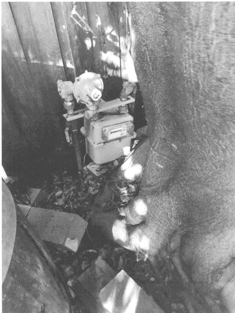
Figure 5: Tree stem expanding into existing services.
