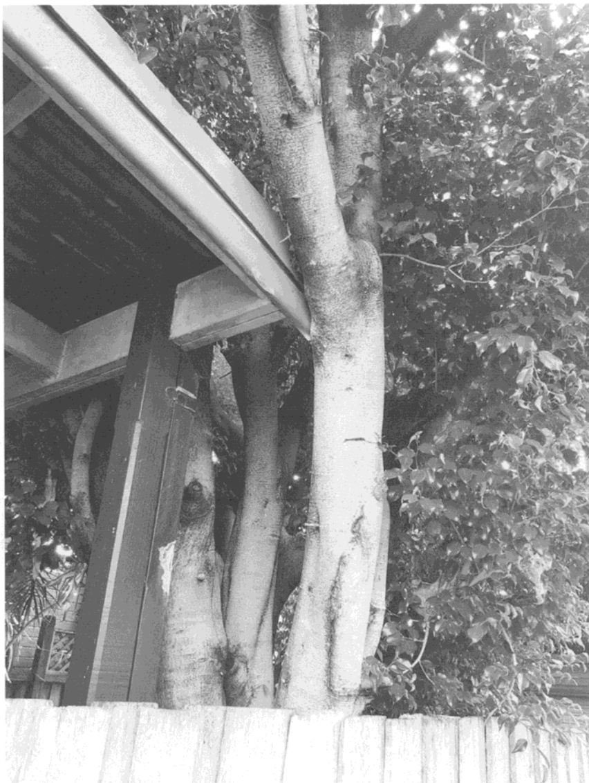
Figure 3 : Damage to fascia that cannot be corrected through pruning.
