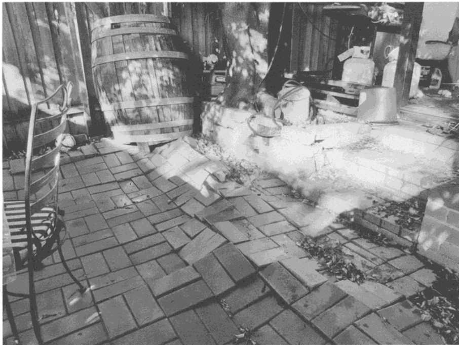
Figure 4; Extensive damage to landscape paving & structures.
