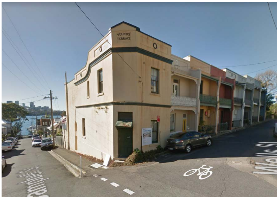
Figure 1: Subject site is second terrace from corner with yellow front door.
