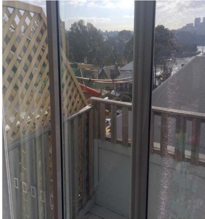
Figure 8: Photo of existing first floor deck balustrading and privacy screening.
