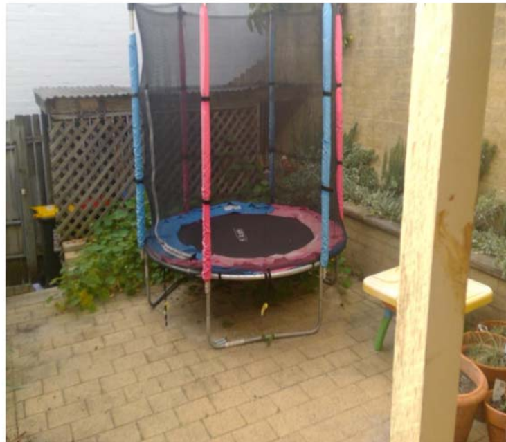
Figure 3: Photo of rear yard, note no soft landscaping that complies with definition of landscaped area.
