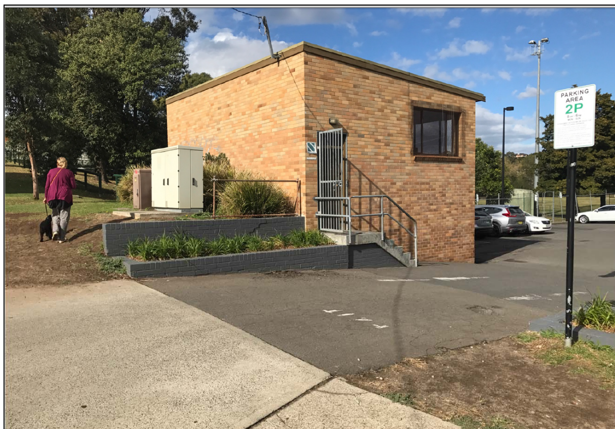
Figure 2 – Existing building viewed from Thornley Street
