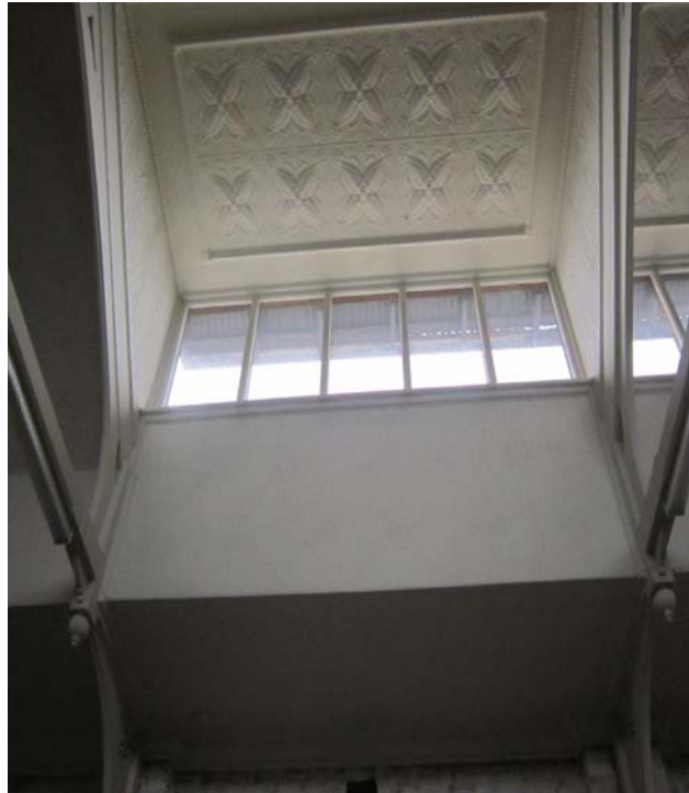
Internal view of existing roof monitor
