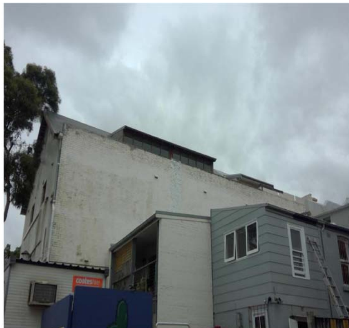
View of roof monitor from Little Darling Street
