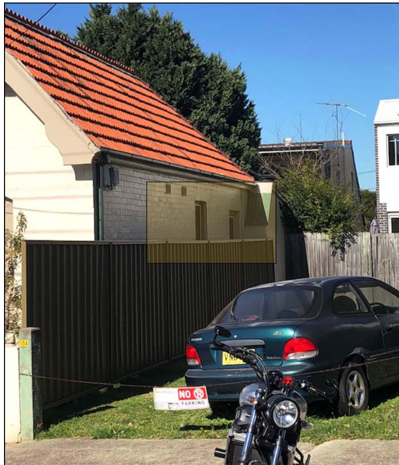
Figure 2: Existing windows of the adjoining property to the north
