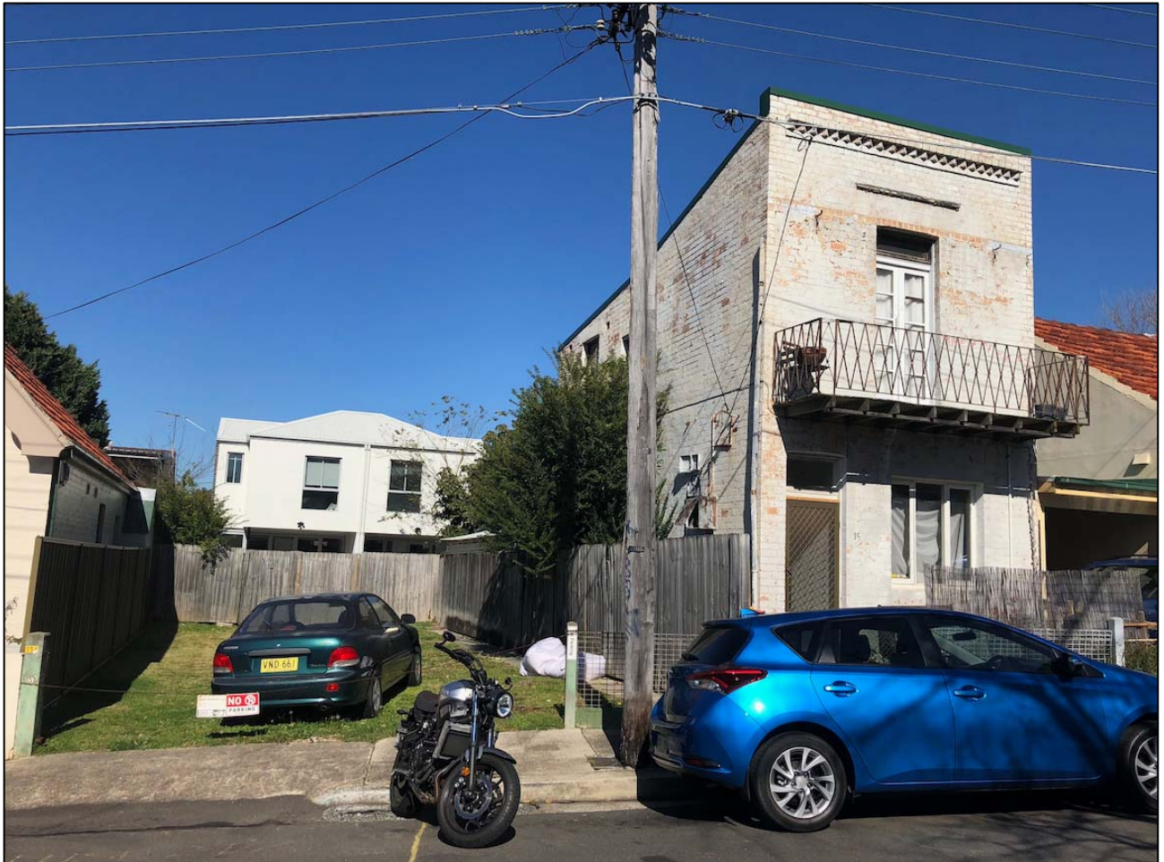
Figure 1: The subject site as viewed from Robert Street
