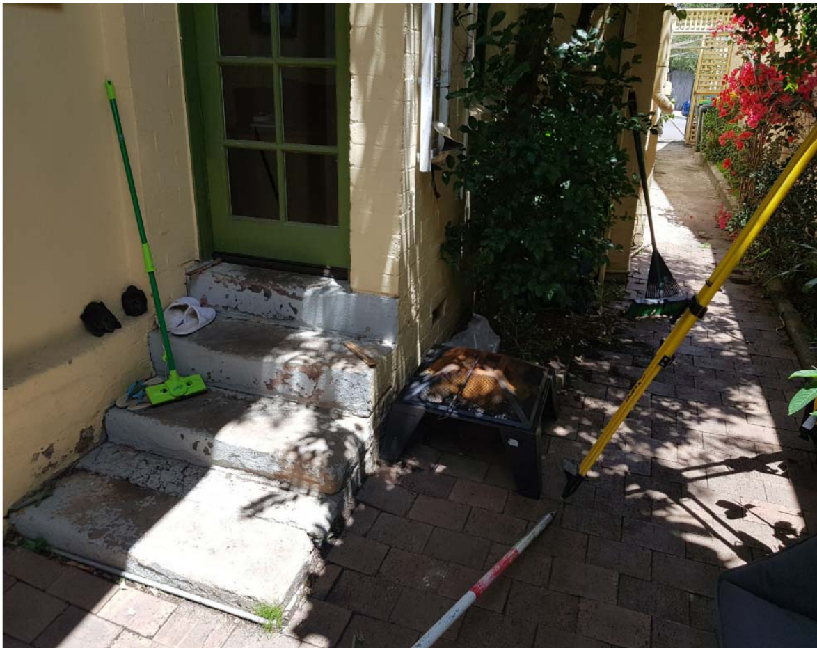
View of Rear of No. 9 Reserve Street
