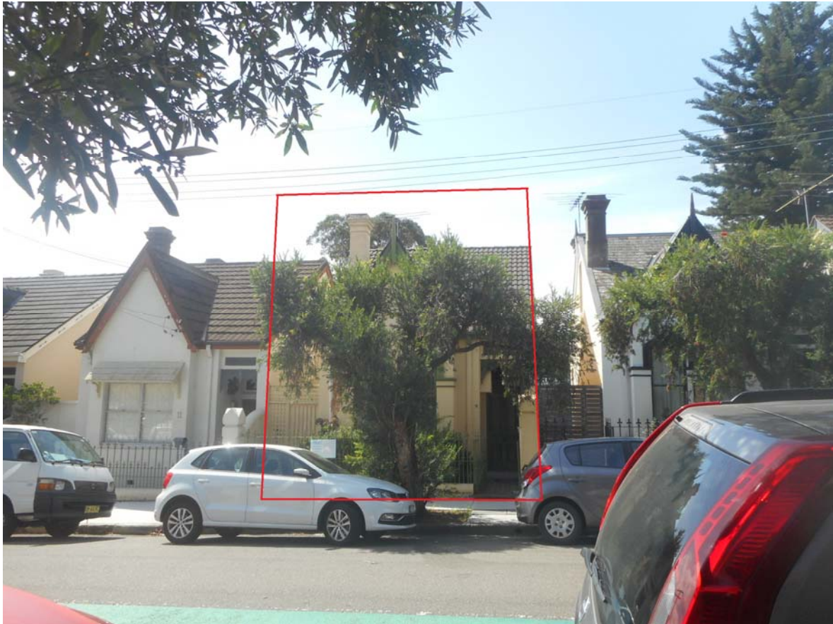
View of No. 7, No. 9 and No. 11 Reserve Street from Reserve Street.
