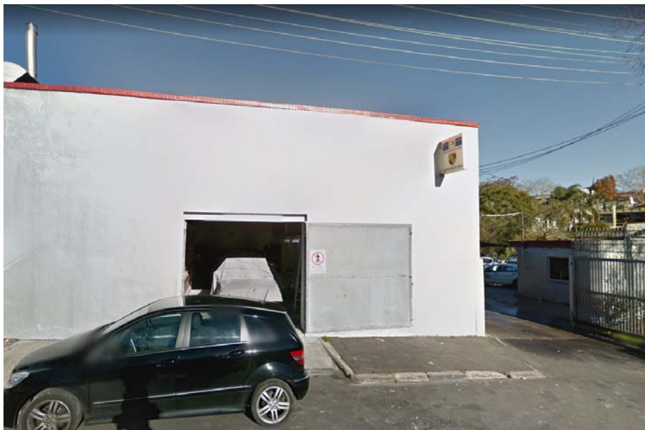
Figure 4 - Existing warehouse when viewed from Chester Street.
