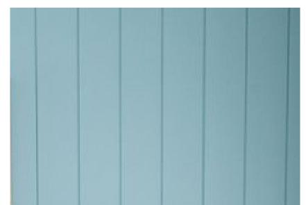
Vertically grooved cladding panels to main building, storage and first aid buildings
