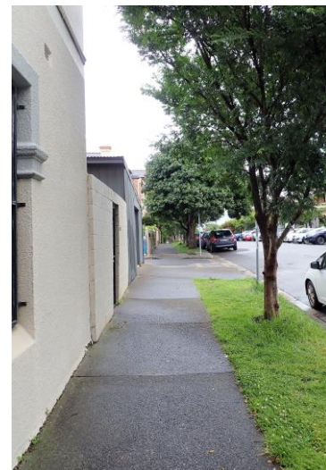
Example of typical concrete footpath with grass verge
