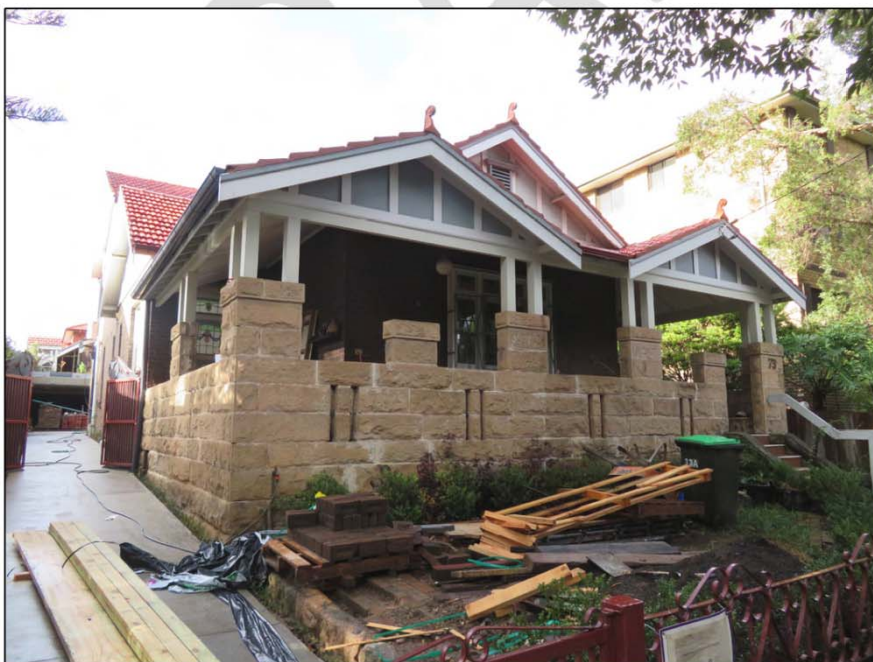
Fig. 4 – Photograph of 73A The Boulevard, Dulwich Hill
