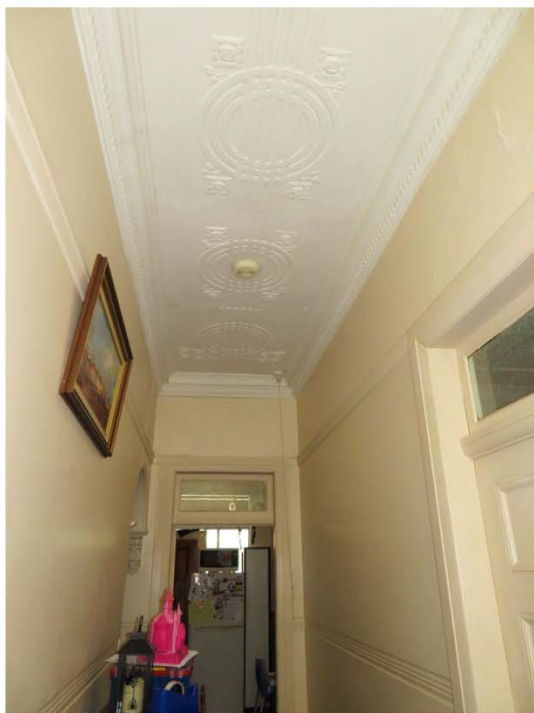
Figure 3.14 No. 73A The Boulevard, Dulwich Hill: Main Hall showing Secession influence on plaster ceiling pattern (Photo: Robertson & Hindmarsh Pty Ltd, 6 June 2018)
