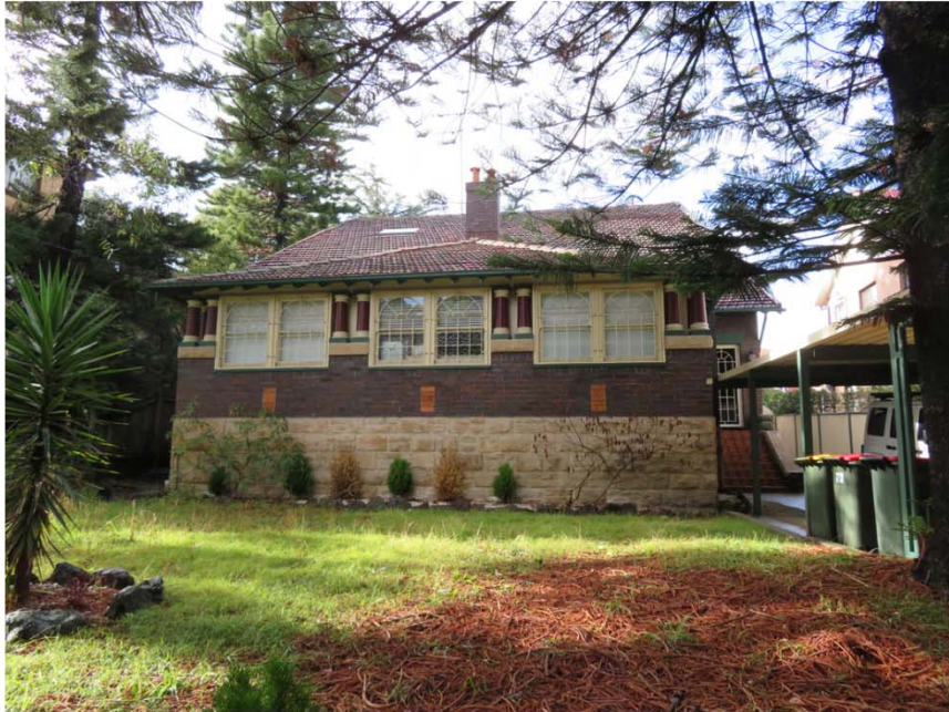
Figure 3.1 No. 73 The Boulevard, Dulwich Hill: Front (west) façade (Photo: Robertson & Hindmarsh Pty Ltd, 6 June 2018)
