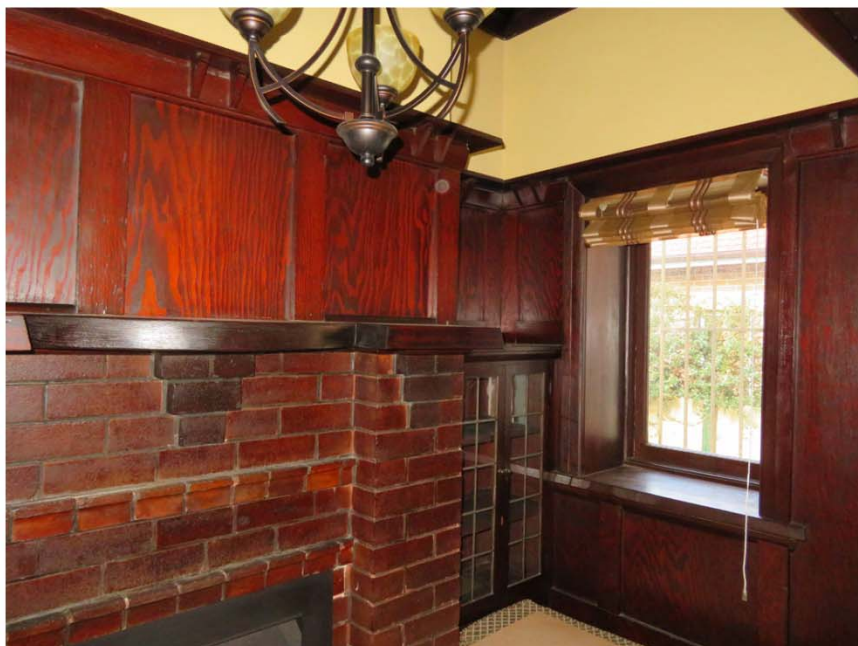
Figure 3.8 No. 73 The Boulevard, Dulwich Hill: Detail of inglenook in Living Room (Photo: Robertson & Hindmarsh Pty Ltd, 6 June 2018)
