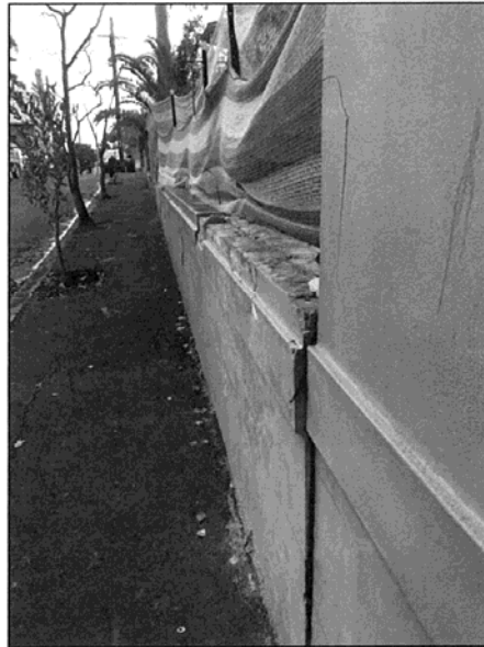
Figure 6: Further damage to retaining wall opposite Tree 2.
