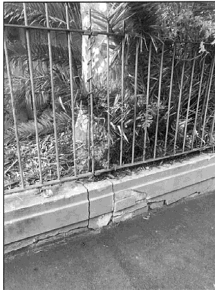
Figure 2: Damage to retaining wall (Tree 1).
