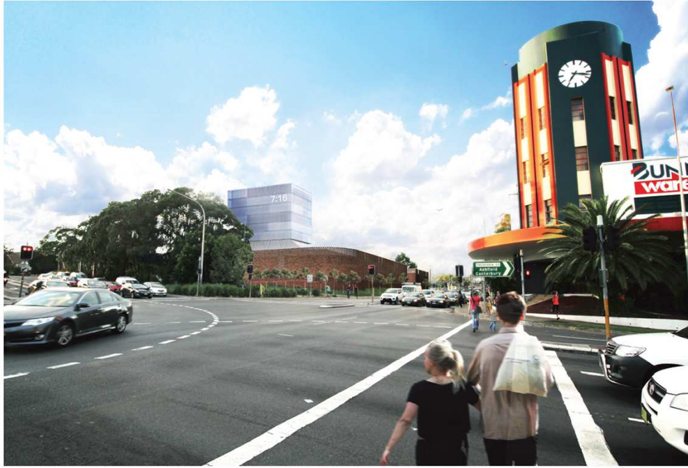
Vent facility at Parramatta Road, Haberfield (Stages 1 & 3) looking north-east
