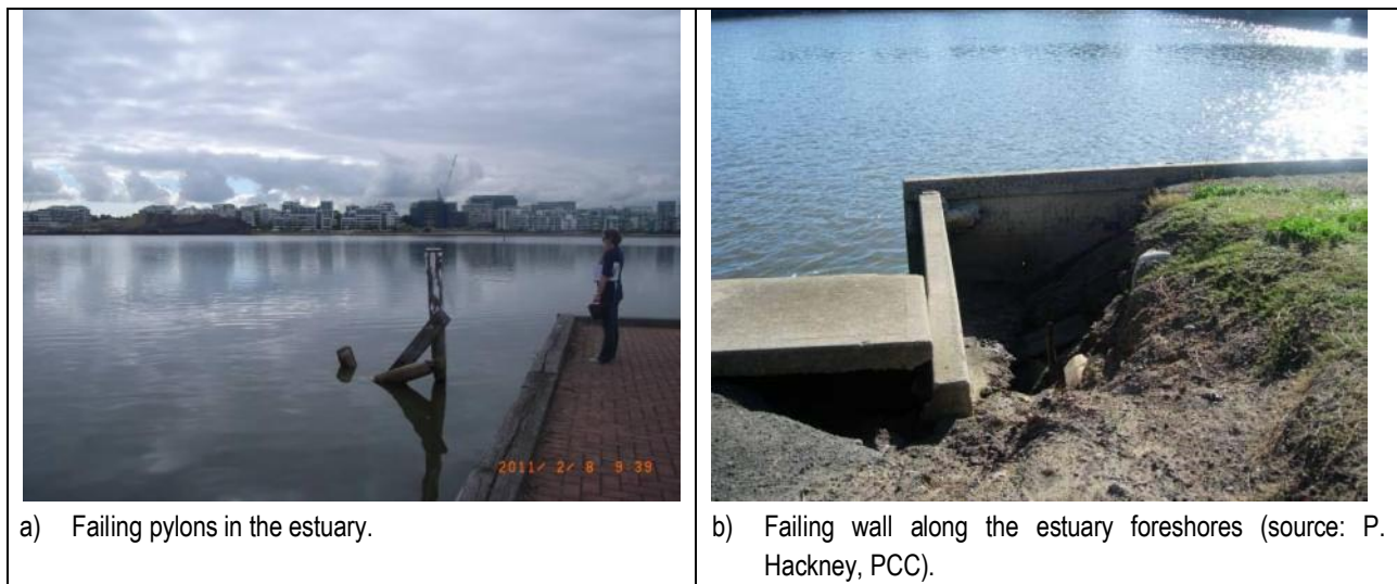
Figure 2.30: Failing Foreshore Infrastructure
