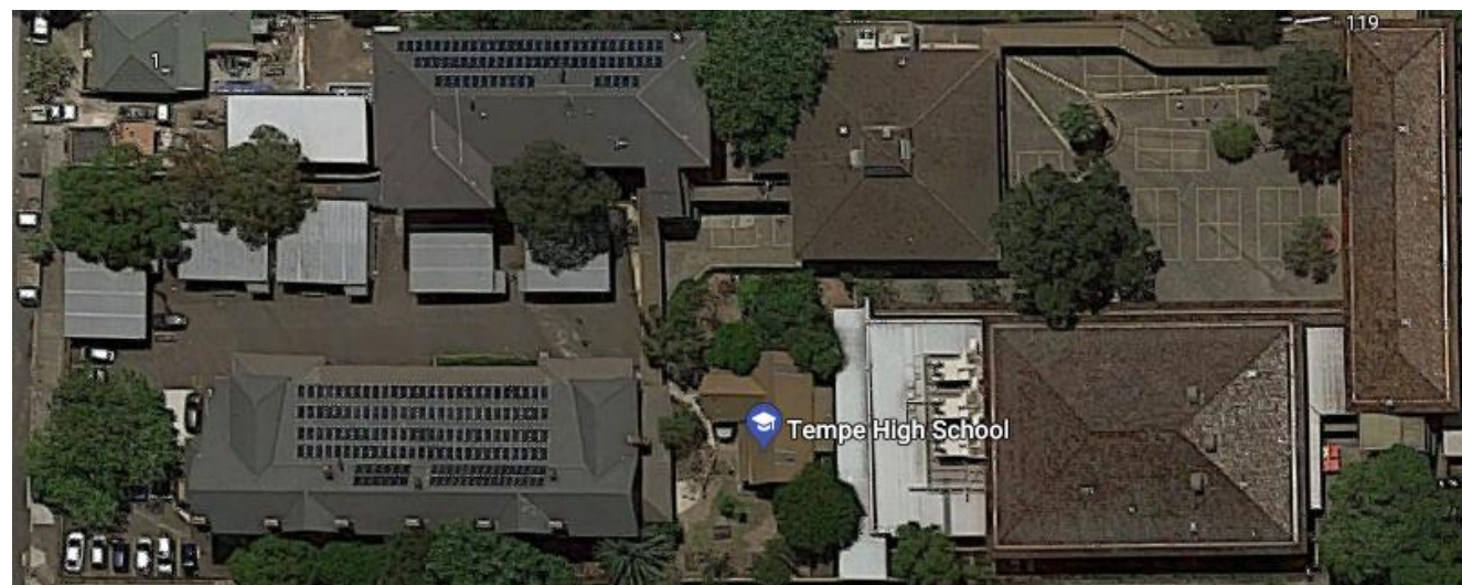
Figure 26: Tempe High School has installed a 50 kW solar PV system as a part of the NSW Department of Education's Resource Efficiency program
