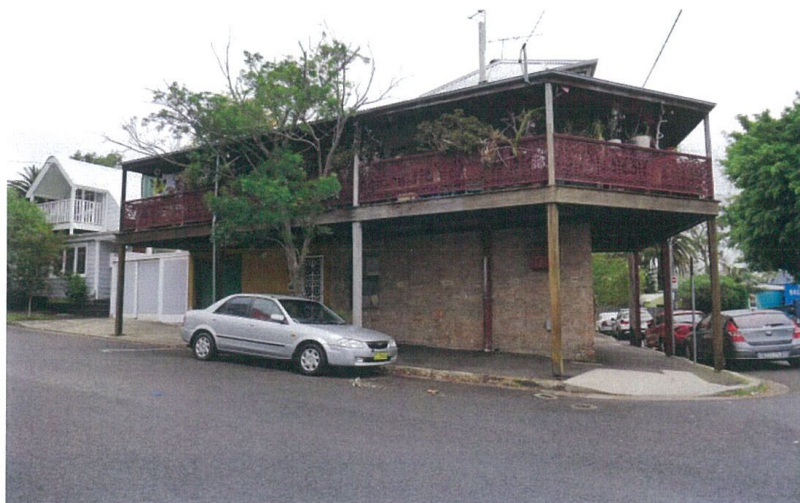
V8 Intersection of Ramsay Street and Smith Street, looking west toward 55-57 Reynolds Street
