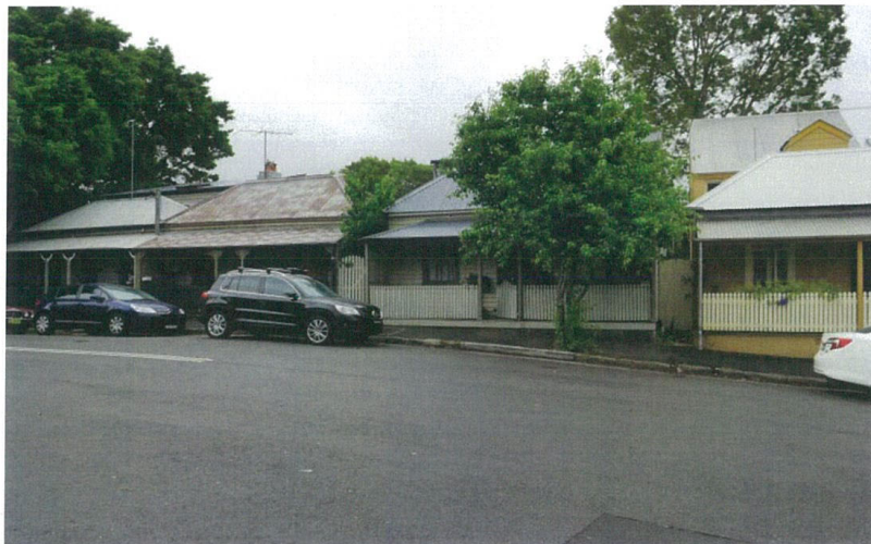
V8 Intersection of Ramsay Street and Smith Street, looking north toward 66-70 Reynolds Street
