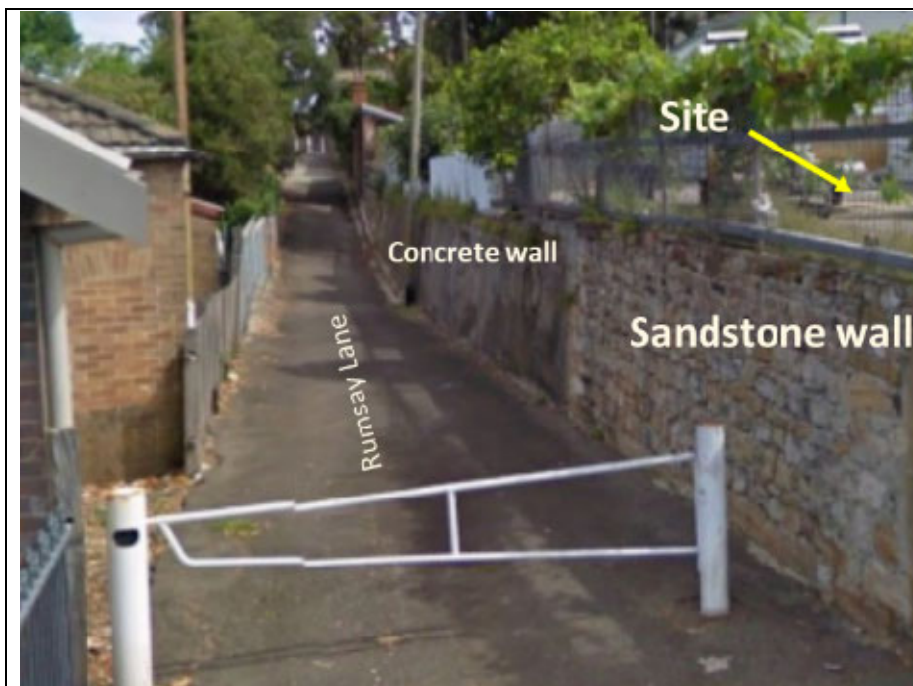
Figure 3: Rumsay Lane to the east of the site and sandstone and concrete retaining wall (Source: Applicant's SEE)
