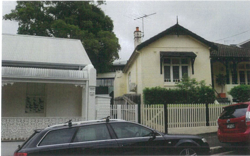
V5 Reynolds Street north of intersection with Foy Street, view west toward site with first floor balcony of 77-79 Smith Street visible between the two houses (63 and 65 Reynolds Street)
