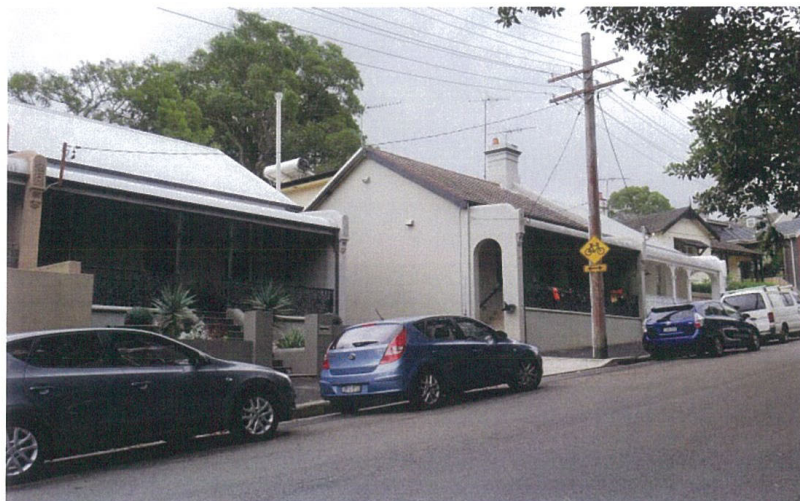
V4 Reynolds Street opposite intersection with Foy Street, view north west toward site
