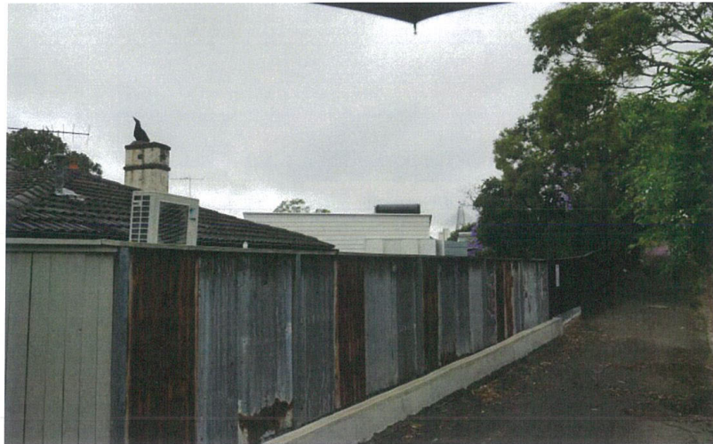
V11 Rumsay Lane, northern section looking south east toward the rears of 61-63 Reynolds Street
