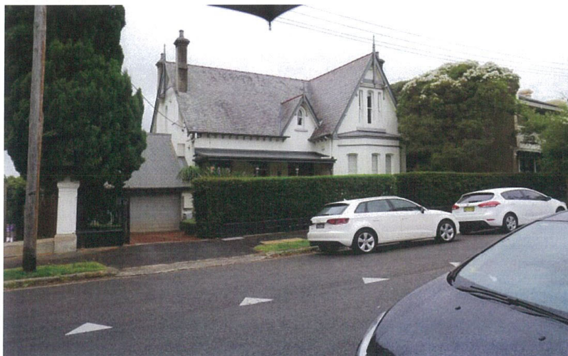
V10 View of 'Providence' 73 Smith Street
