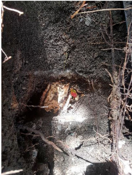
Fig 5. Photo of 100mm Ø tree root and root matrix in excavation .
