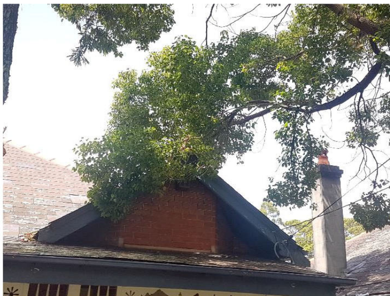
Fig 10 Photo of limbs in contact with Mr. Zhang's roof.
