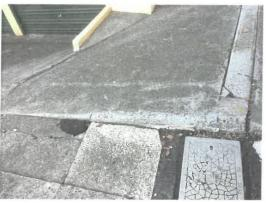
Figure 5 Concrete lifting at driveway entry.
