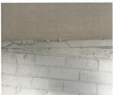
Figure 8 Cracking of walkway from brick wall.
