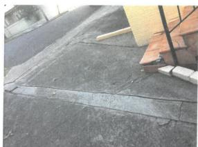
Figure 4 Concrete strip showing repaired sewer
