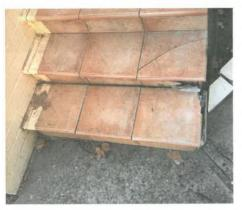
Figure 9 cracking of lower two stairs.
