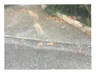
Figure 7 Concrete lifting, entry to laundry.
