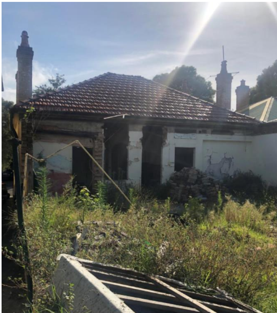
Figure 2: Rear of remains of existing building
