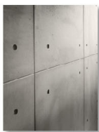
'P6' – Concrete Panels Wall cladding - Lift /Entry Canopy/ Feature Wall
