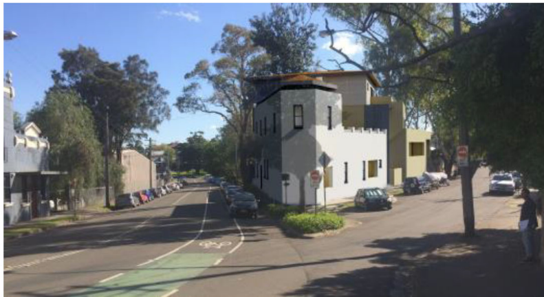
View of the intersection of Lilyfield Road and Burt Street
