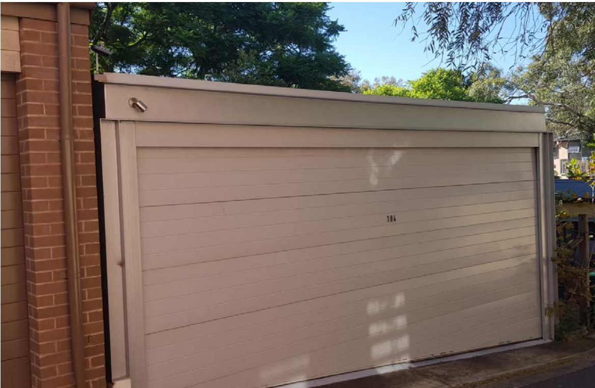
Figure B. Existing garage with existing steel beam exposed.
