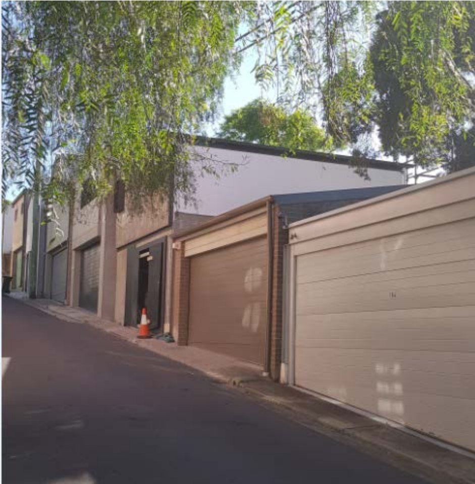
Figure C . Existing view looking north-east towards 184 Nelson Street Annandale.
