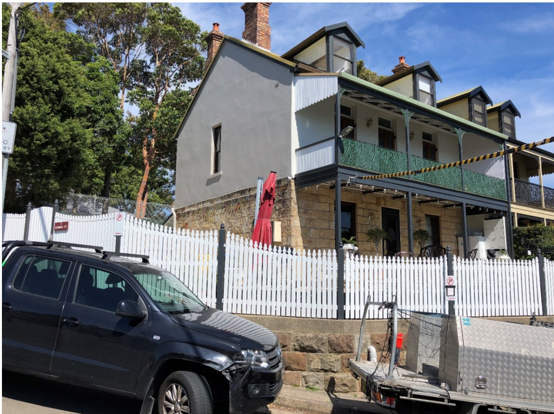
Picture 2 Site Photo – School Street frontage
