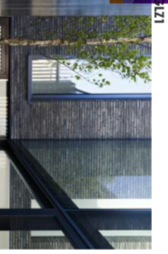
GLZ1 CLEAR GLAZING IN ALUMINIUM FRAME FINISH TO FRAME SW/EGC TO G. JAMES ANODOSED 'BLACK SLAVE'
