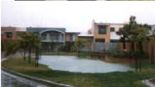
Infiltration basin under normal conditions (above), and during heavy rain (left).
