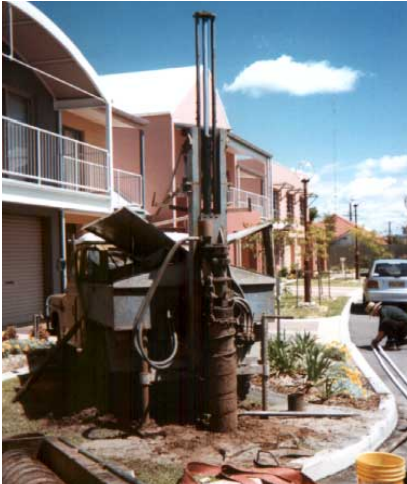
Installing a groundwater bore
