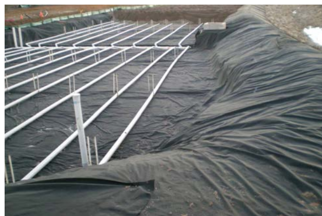
Figure 20 Bioretention system liner extended over embankments
