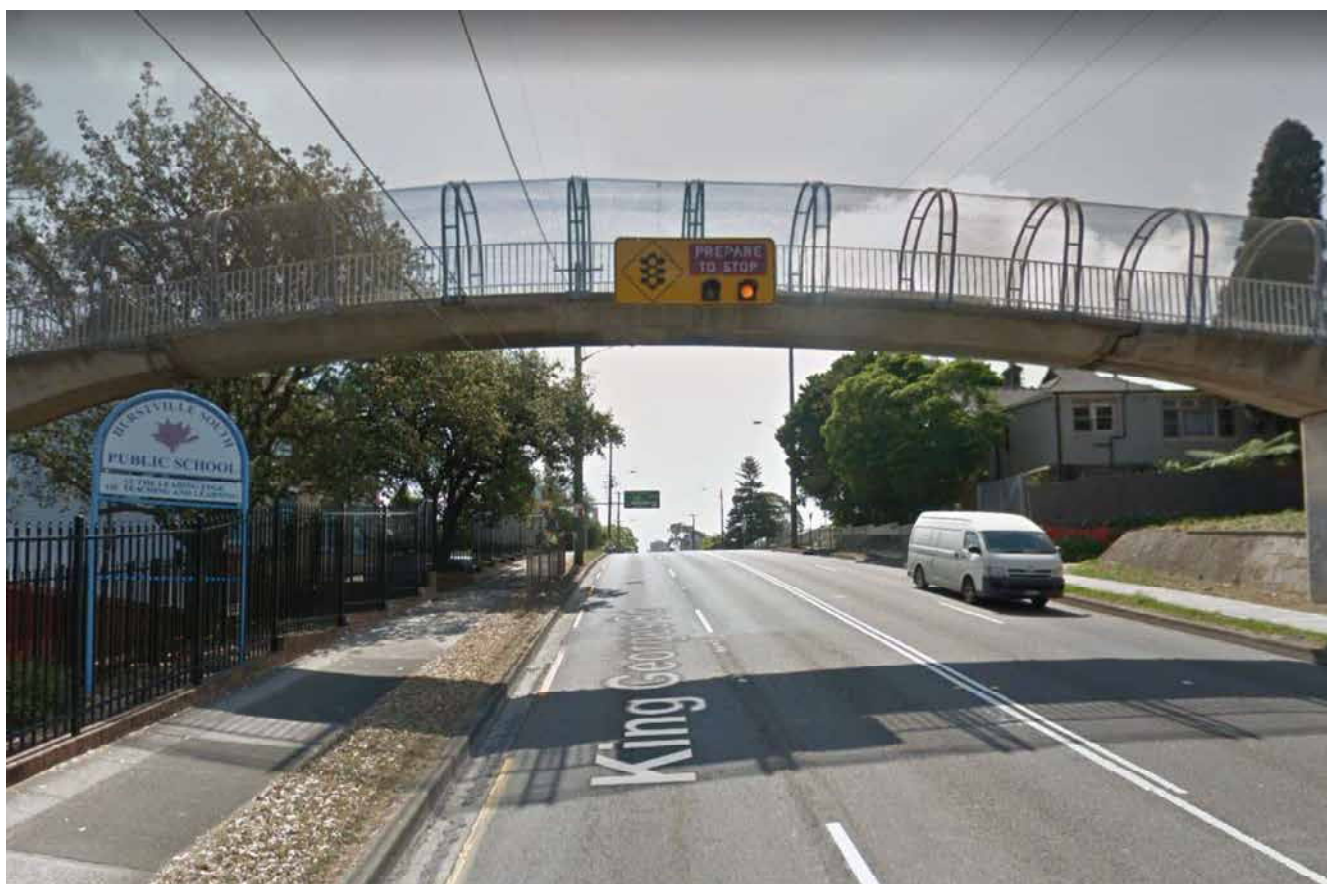
Figure 5.16 : Wig-wag warning sign (King Georges Road near Hurstville South Public School, Hurstville)
