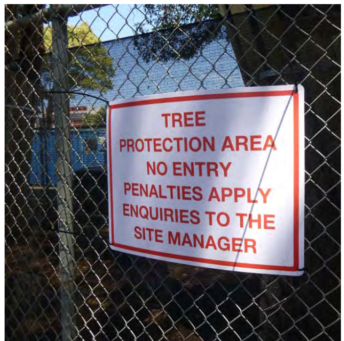
Figure 2.28 - Depending on the nature of the development Council may also require suitable temporary tree protection fencing and signage (Photo: Arterra)
