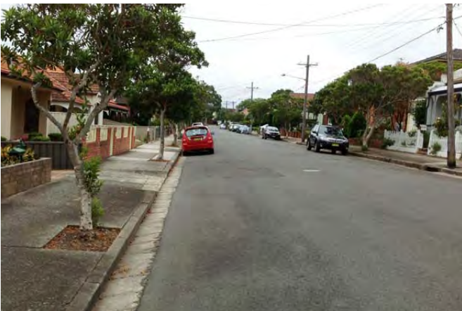
Figure 1.34 Typical fully-paved verge with tree planting, Dougan Street, Croydon South (Photo - Arterra)
