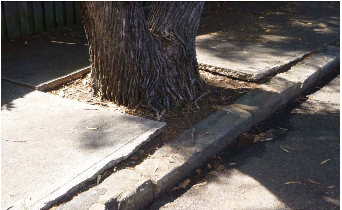
Figure 2.6 - Although street trees have many benefits, large trees can also often cause disruption to surrounding infrastructure, particularly when they are planted close to kerbs and guttering. This can also cause disruption to drainage and lead to further road degradation. In quiet streets this can often be rectified through kerb extensions or the creation of rain gardens and the like, while still retaining the tree. (Photo - Arterra)
