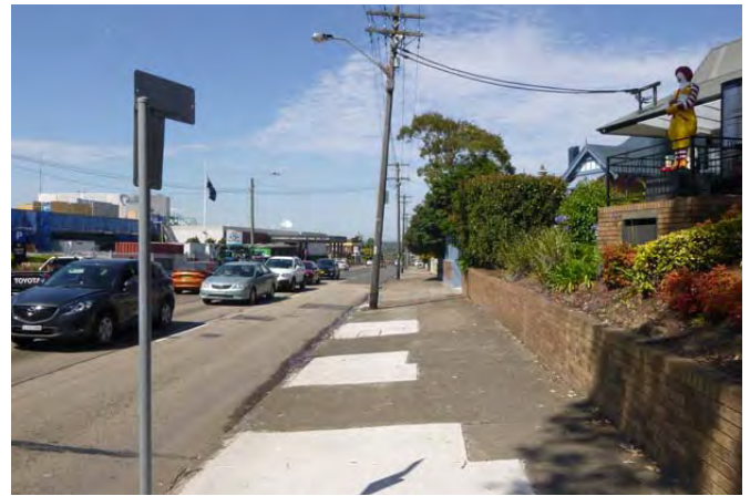
Figure 1.25 Canterbury Road, Hurlstone Park - commercial development (Photo - Arterra)
