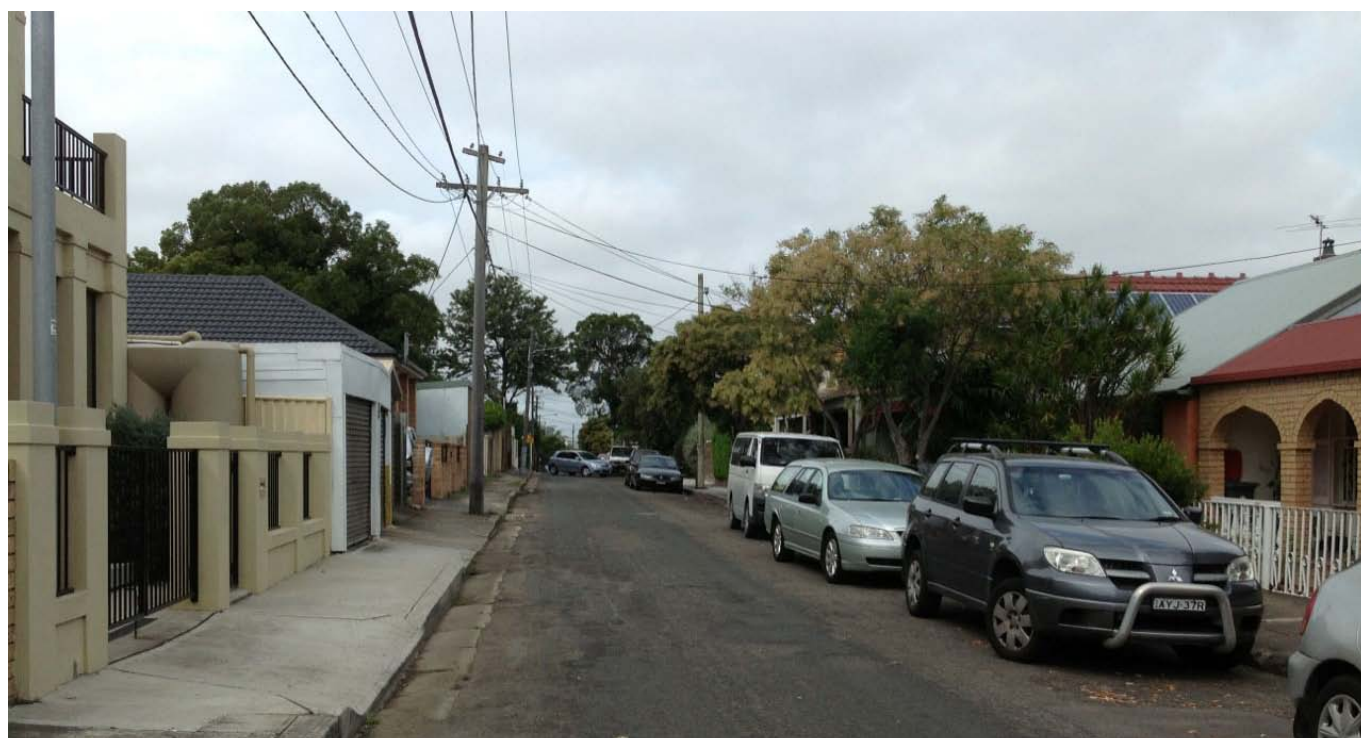
Figure 5.23- Many streets have narrow footpaths and overhead wires and tree planting is difficult, for example in Edith Street, St Peters (Photo Arterra)
