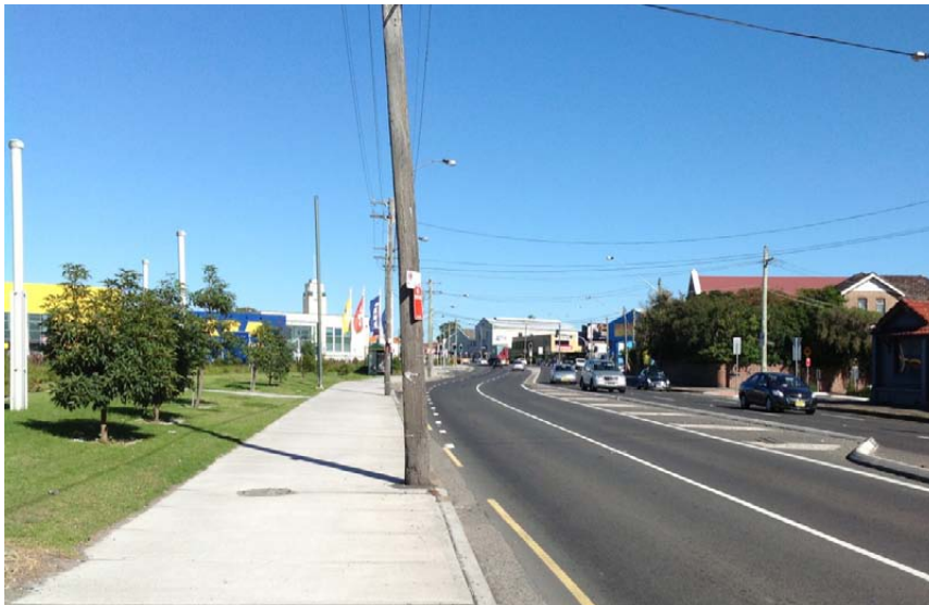
Figure 4.4- Existing - Princes Highway, Tempe.
