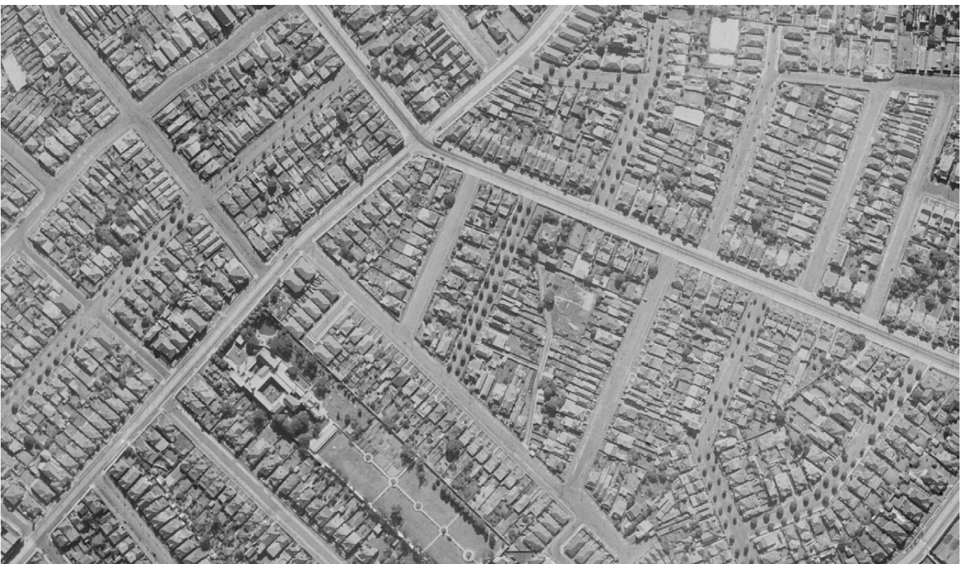
Figure 1.4- View over Marrickville in 1943, with the tree planting in streets like Canonbury Grove, Woodcourt Street, Robert Street and David Street clearly visible. Most other streets had very little if any street tree planting until much later. (Source: NSW Lands Dept Six Viewer)
