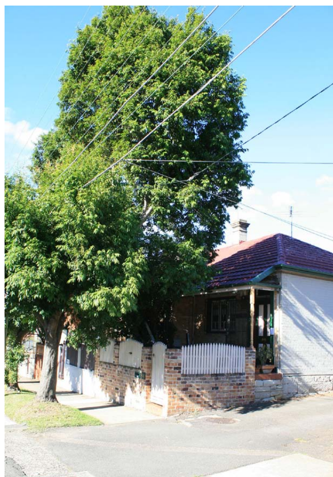
Figure 1.15 - An example of excessive overshadowing on the south side of a street with small building setbacks and impact with overhead wires (Photo Arterra)
