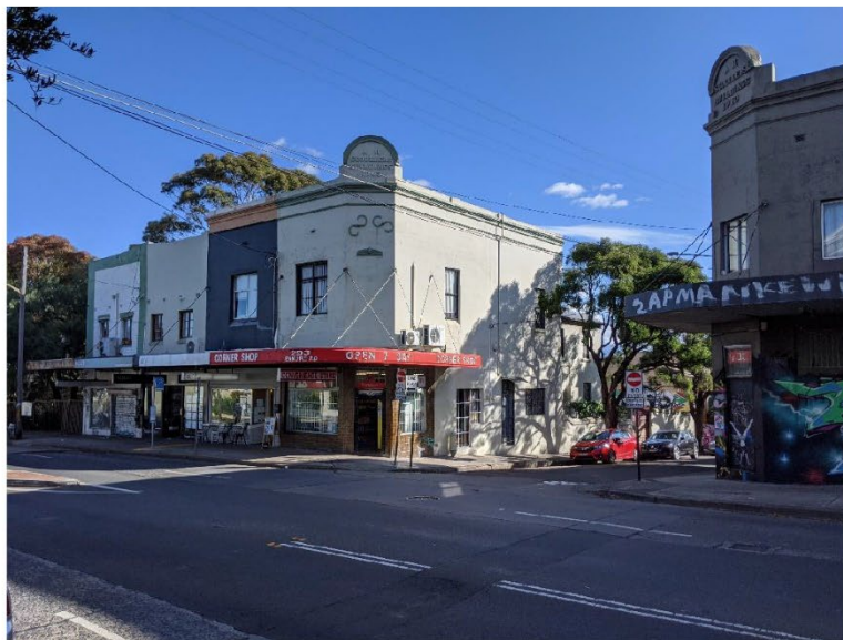
Figure 6: View of a pocket of E1 zoned land at 299 (far left) to 291 (right) Enmore Road
