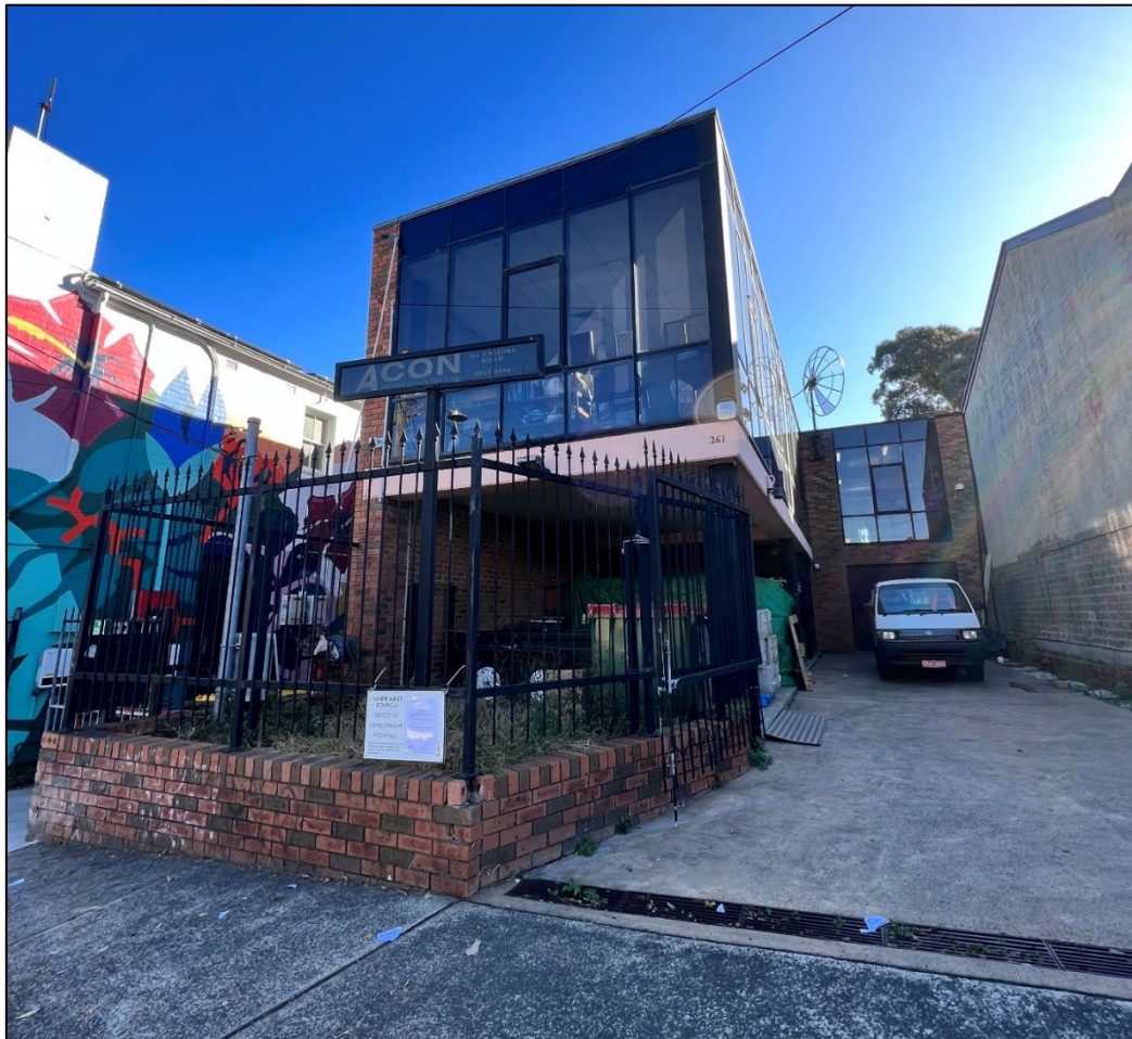
Figure 3: Photo of the subject site when viewed from Enmore Road.
