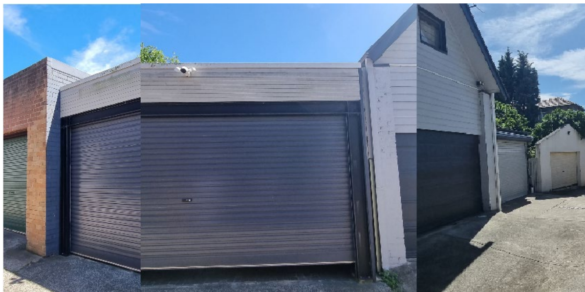
Rear of subject site
