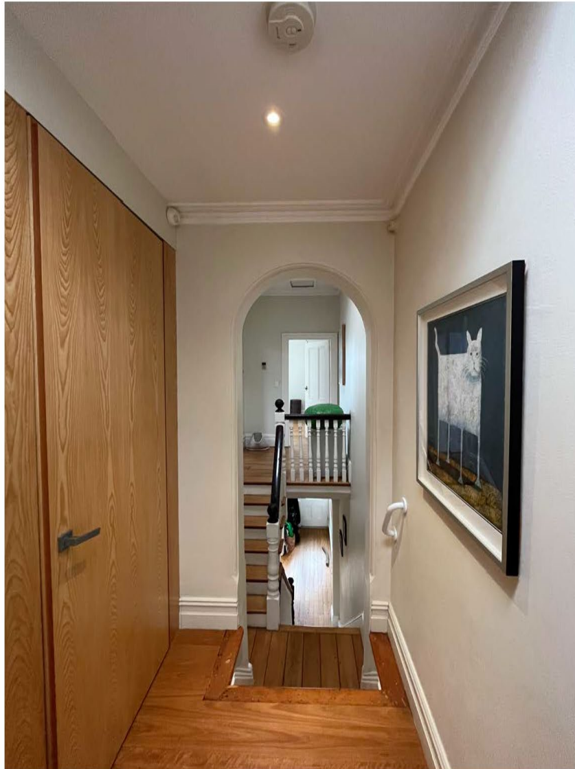
Figure 20: Existing second floor split level staircase. The proposed staircase for the attic is to be located on the right attached to the party wall.
