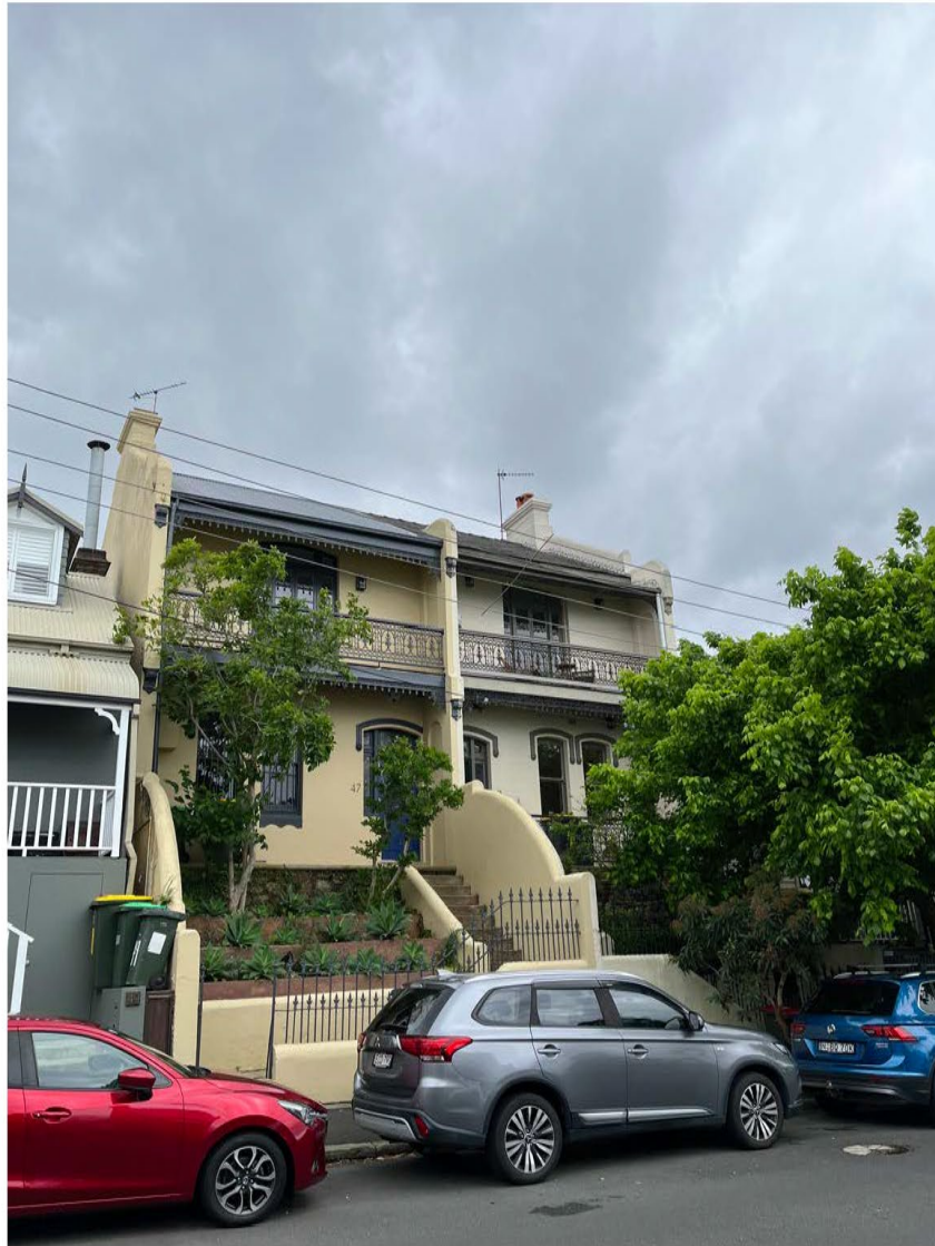
Figure 16: 47 and 45 Bradford Street.
