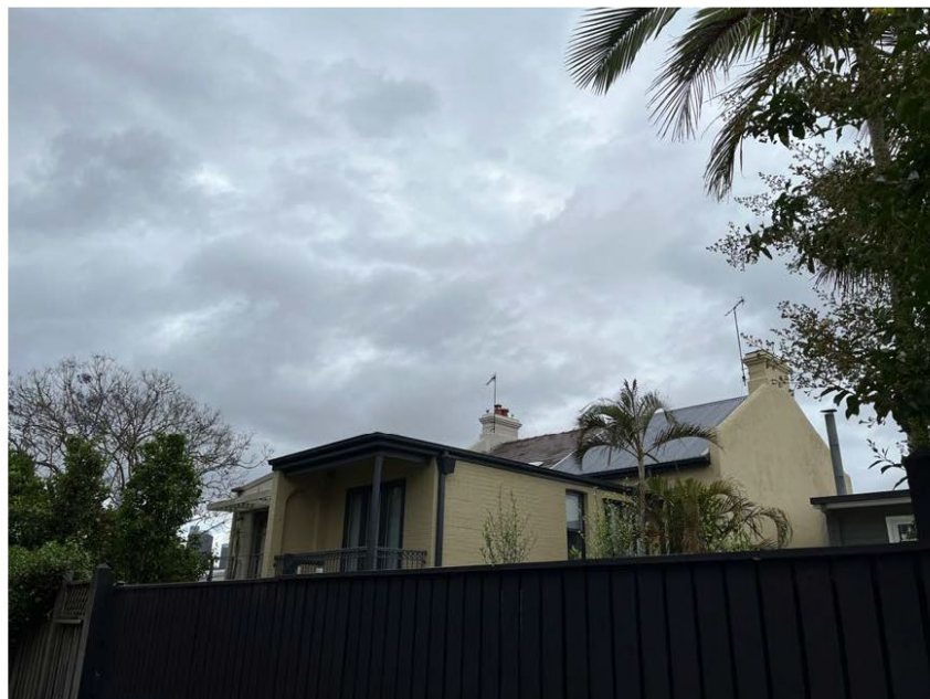
Figure 18: No 47 and 45 Bradford Street, viewed from Bradford Lane.
