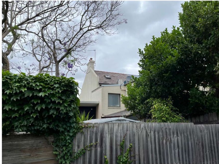
Figure 17: No 45 Bradford Street viewed from Bradford Lane.
