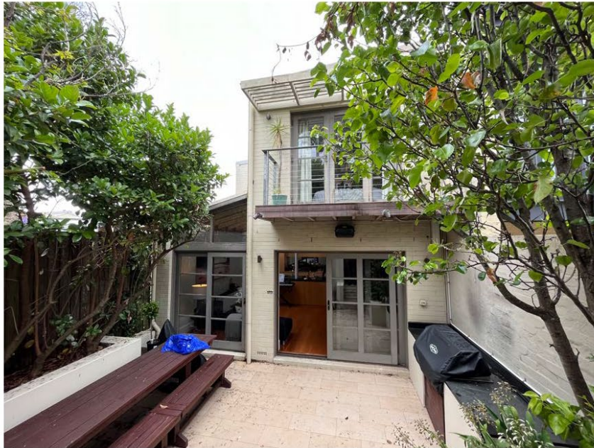
Figure 19: View from the backyard looking south at existing Family Room and Bedroom 4 on the first floor with balcony.
