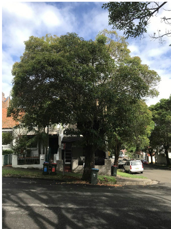
Figure 3: Photo of subject site
