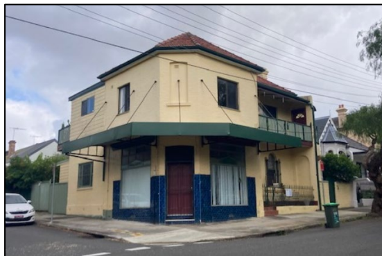
Figure 3: Photo of the subject site (as viewed from the south east on Moonbie Street).
