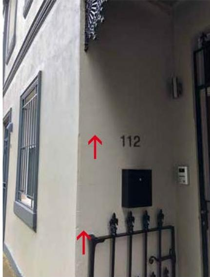
**Figure 8** | *Traces of ashlar scribing on the side. The front elevation was rendered recently with smooth render.*
