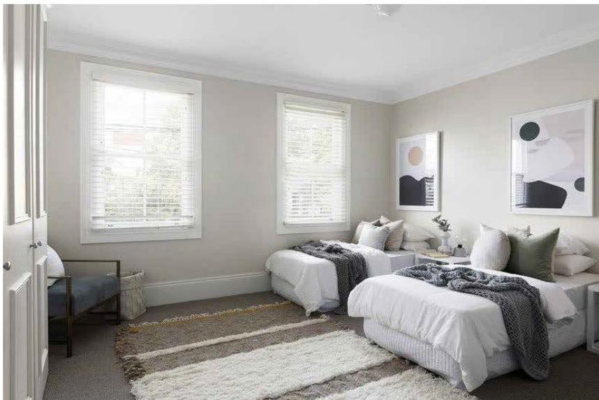
**Figure 16** | *The front bedroom. Note the poorly detailed architraves: there is no sill piece.*
