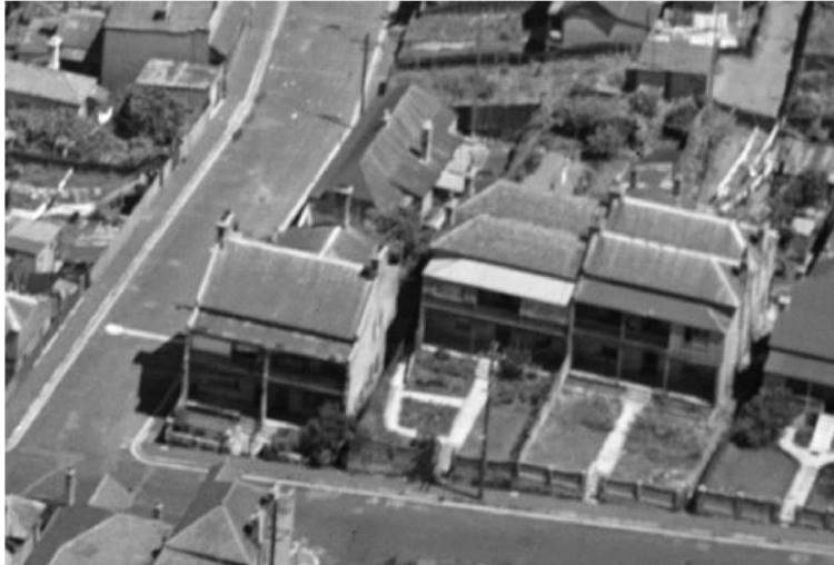
Figure 2.6 The Jane Street frontage of Nos. 15-17 in either the 1930s or possibly early 1950s Source: State Library of NSW (c112370002)
