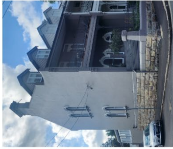
EXISTING HOUSE RENDERED MASONRY STONE BASE TERRACOTTA TILE ROOF COLORBOND ROOF SHEETING STEEL PALISADE FENCE
