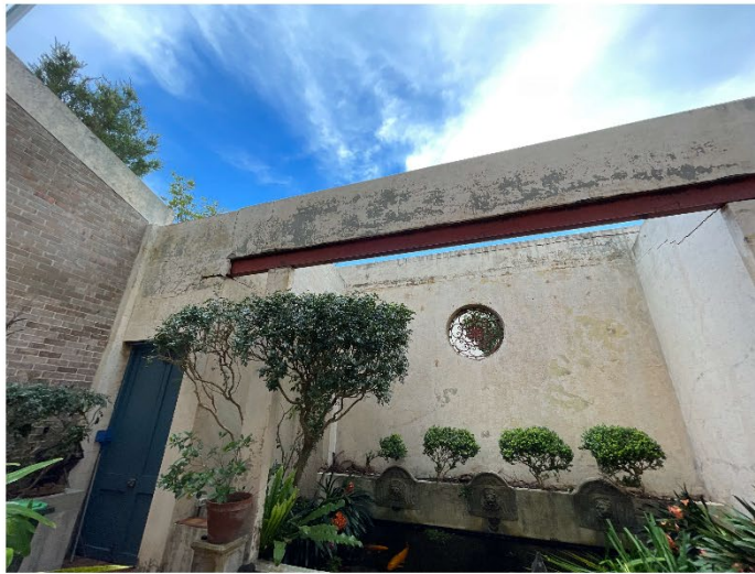
Figure 14. Courtyard with ivy removed 2022 (Source: Structural Report by Luff Pier Engineering)
