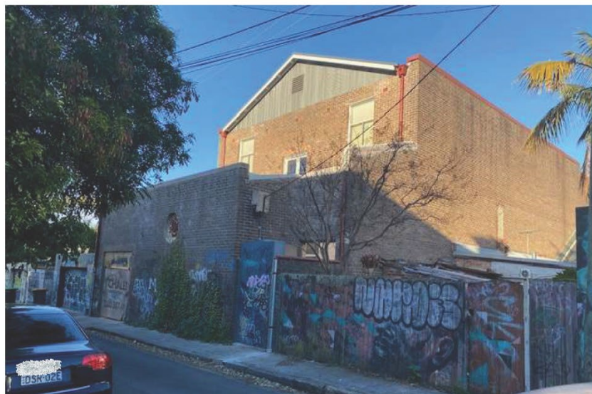
Figure 4. Rear view of the site from Bailey Street
