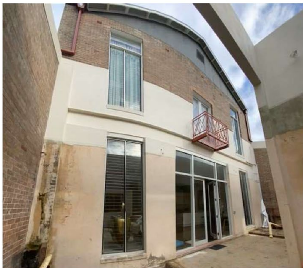
Figure 14. Remedial works completed (July 2023)
