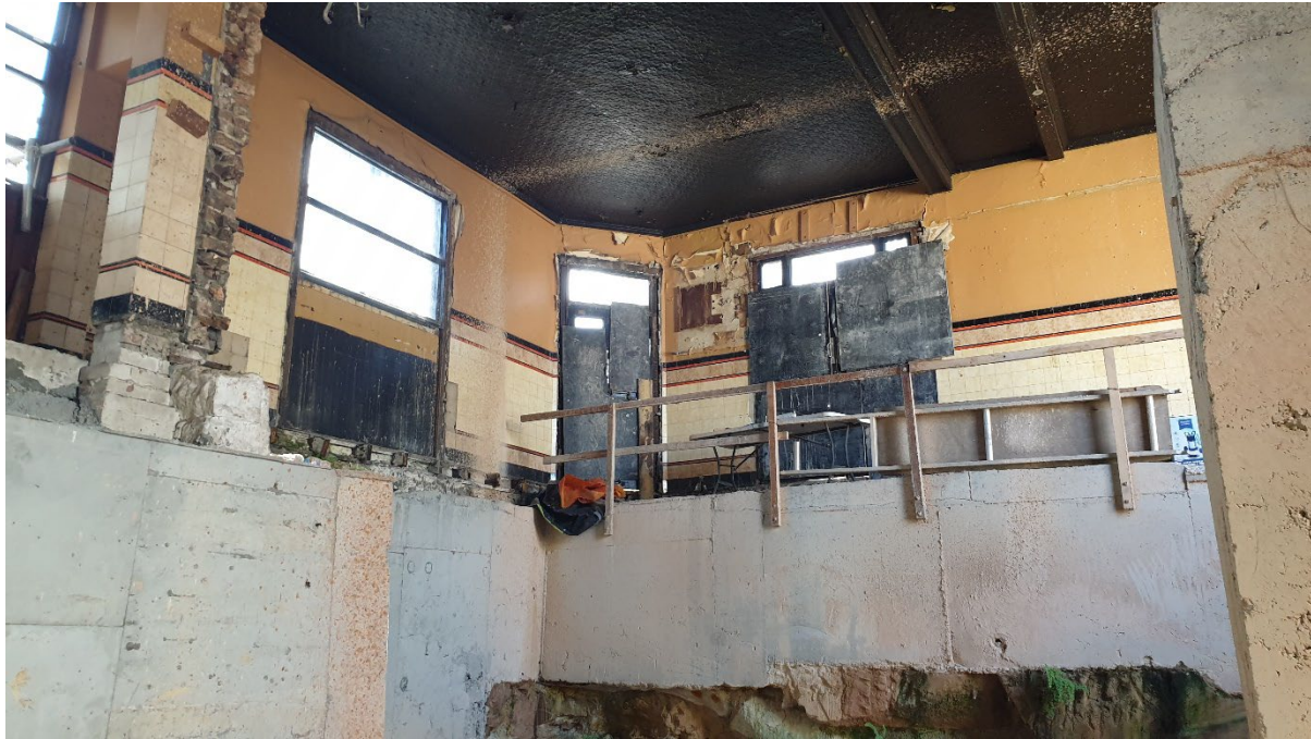
Photo of current site conditions inside the pub area
