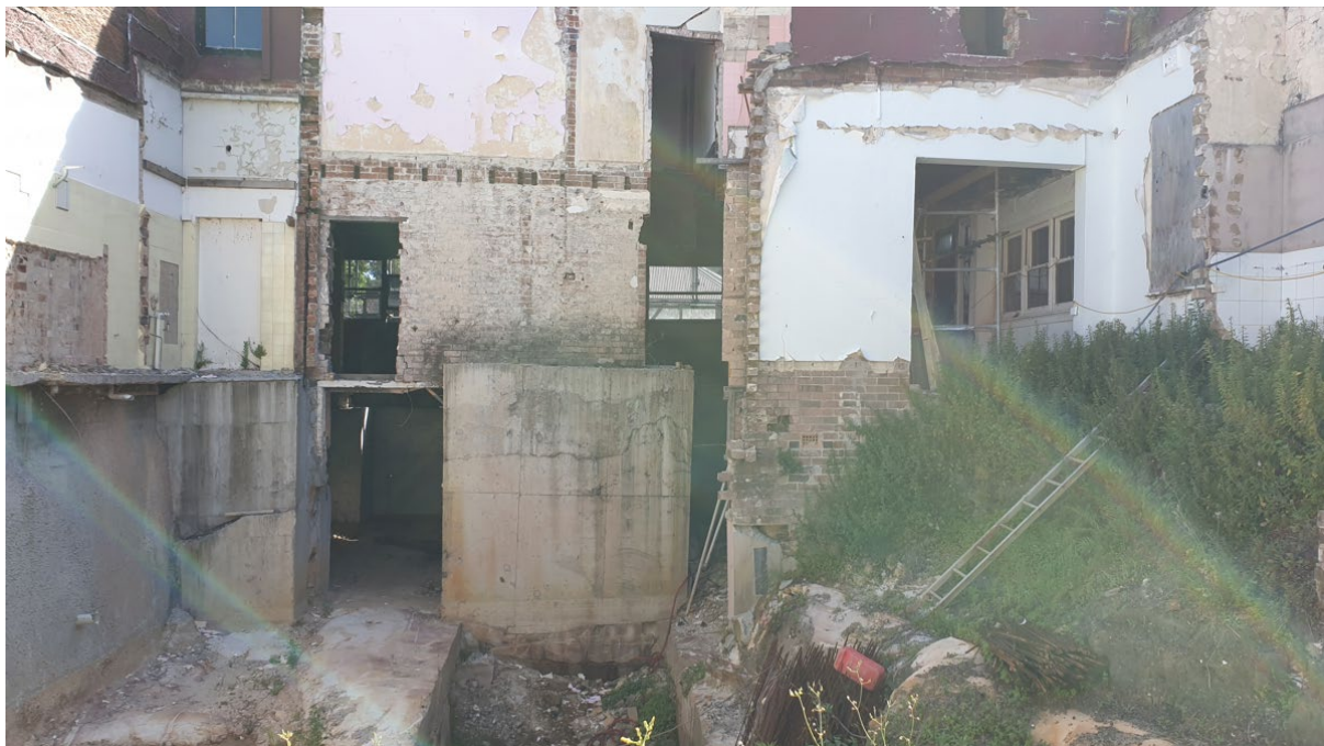
Photo of current site conditions
