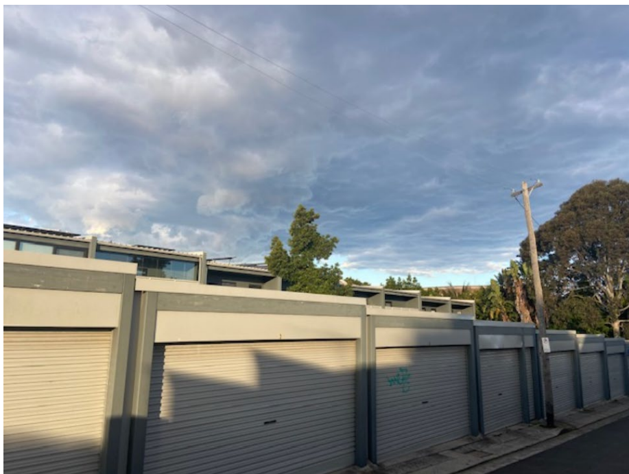
Figure 2 - Image of the carports of the attached terraces fronting Lynch Lane.
