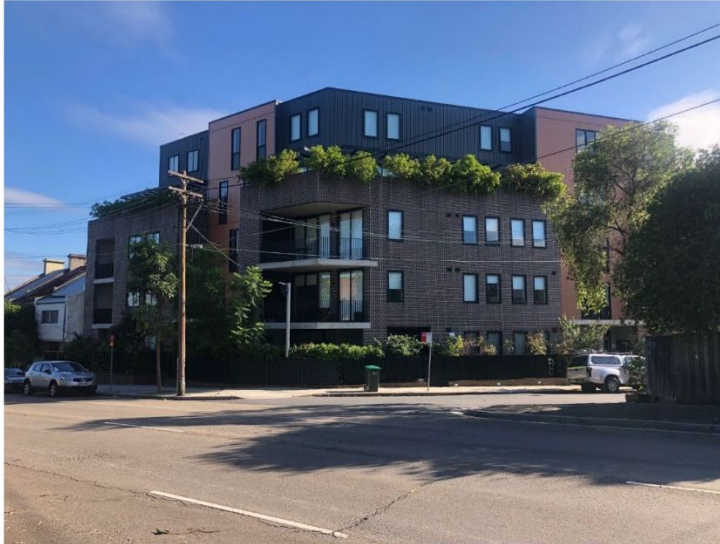
Figure 4: Five-storey residential flat building at 20 Sadlier Crescent
